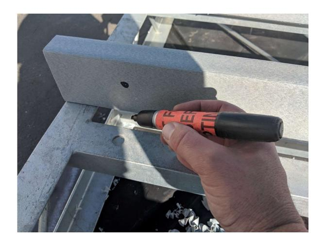
Using a small drill bit, drill through the board at the sharpie mark. Once pilot hole is drilled flip board over, use a paddle bit and drill  $\frac{1}{4}$ " or so down to recess the Carriage bolt head.
