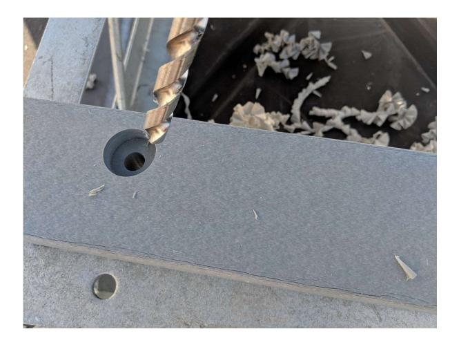
Once holes are drilled, bolt sleepers to the frames using the 2.5" carriage bolt sets.
