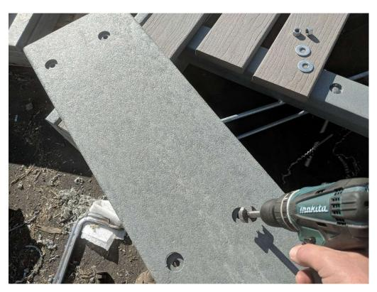
Bolt the fascia boards to the frames using the 2.5" carriage bolts.
