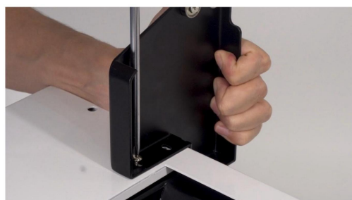
Step 5. Put the bracket on and pay attention to its facing direction. Turn the screws but do not tighten it fully.
