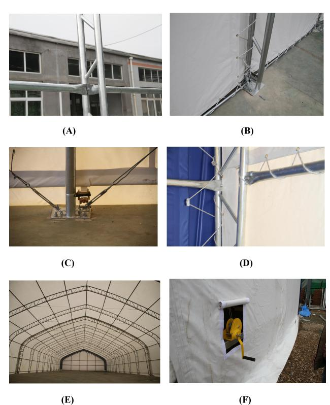
NOTE: DO NOT LEAVE THE ROOF COVER UNATTACHED UNDER ANY CIRCUMSTANCES until the final assembly and tightening has been completed. The process is quite easy. But some tightening adjustments will be necessary to produce a flat, tension ed roof cover. Please adjust the roof cover every month.
