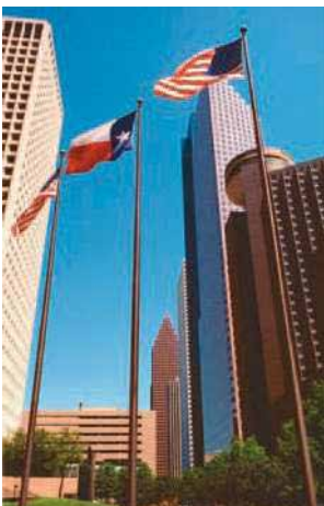
Allen Center (below) Three 70 ft. Aluminum Flagpoles and 12x18' Flags.
