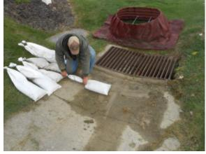
Fill sandbags (provided) half full with sand or gravel so they will lie wide and flat. Optimum thickness is 2" Note the long apron in front of the grate. Large concrete aprons can double or triple the cost of installing 2x4s and silt fence around the perimeter of the grate.
