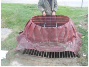
Position the SedCage over the grate and center it. Extend geotextile flap out around SedCage. The camber of the SedCage matches up with the pitch of the grate.
