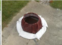
ODOT Catch Basin No. 5 and the SedCage "SC-42-sand". Note the amount of the 2x4 and silt fence method that would have been required due to the large concrete apron.
