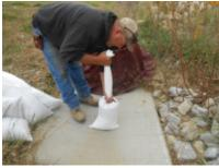
Fill the provided sandbags half full with sand so they lay wide and flat. Optimum thickness is 2". Surround the SedCage with the sandbags.
