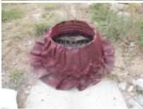
Position the SedCage over the grate and center it. Extend the geotextile flap out around SedCage.
