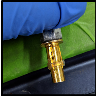
Next apply silicone to the plusnuts before inserting to insure a water tight seal
