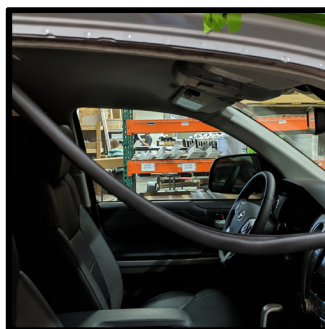
Pull back the door trim to remove any metal shaving that fall thru while drilling
