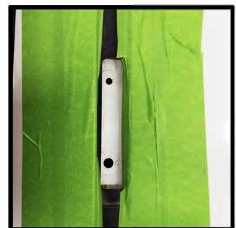
View of bottom hole drilled, be sure to clean any shavings away that fell thru while drilling.
