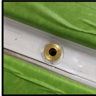
Insert into the roof.
