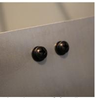
Complete step 3 for all ten mounting holes on the the wind deflector. The correct order is screw, lock washer, flat washer, deflector, tnut. The screw should be loosely threaded into the tnut.
