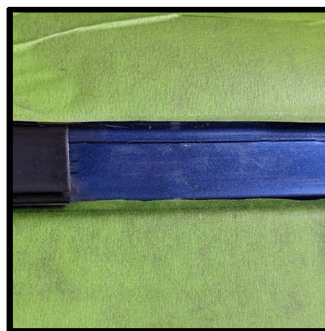
Trim removed and foam tape cleaned away
