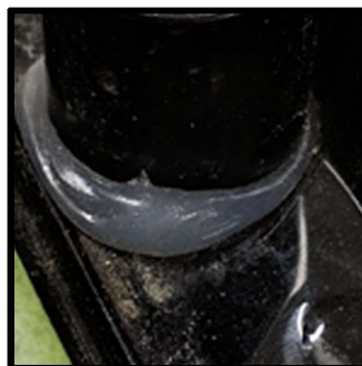
Before placing the spacers down apply a liberal amount of sealant to ensure a water tight seal
