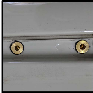
Plusnuts in roof
