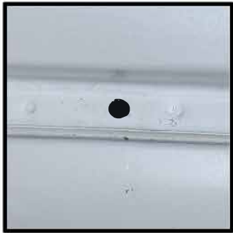
Hole cleaned out to 3/8"
