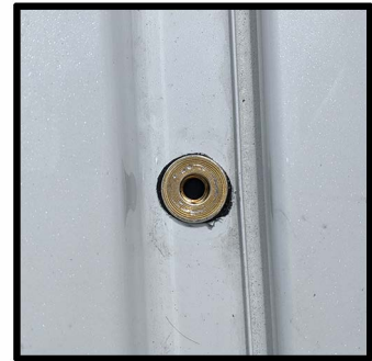
Plusnut placed in roof
