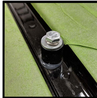
Apply more silicone and place the spacer on the roof.
