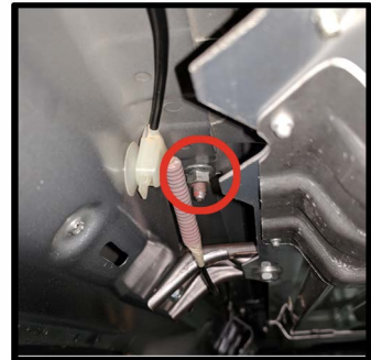
There are 5 five nuts that need removed to remove the roof rails
