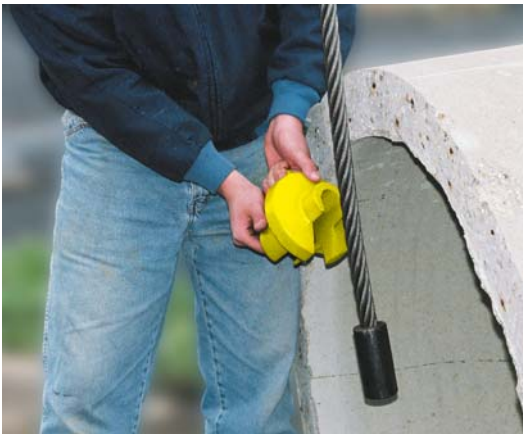
Drop pipe carrier lifting sling through hole in pipe. Align and insert “Tea Cup” pipe carrier into lifting sling.
