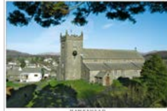
DP707 Hawkshead Parish Church
