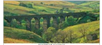
WH030 Denthead Viaduct
