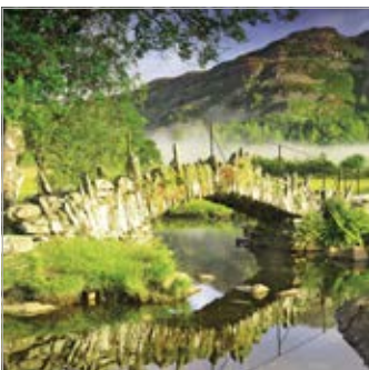
LMG040 Slater Bridge, Little Langdale
