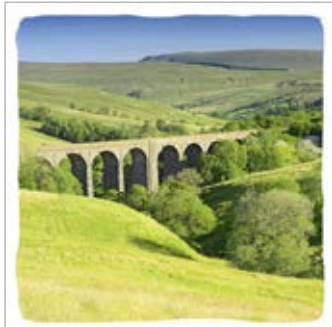
VGD005 Dent Head Viaduct
