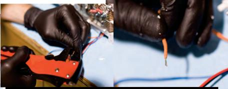
22 Cut the wires to a reasonable length and strip the ends. We'll only be cutting the orange, red and black wires for now. Using an appropriate wire stripper (whatever you've got laying around can make due), strip the ends of the wires that will be going into the connectors.
