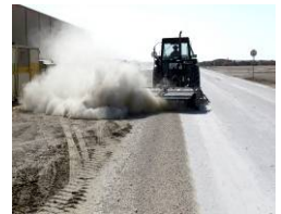
Road Shoulders Shoulder Dust Control Shoulder Erosion Control Shoulder Stabilization
