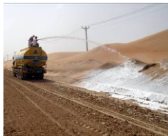
Slopes & Berms Slope Erosion Control Slope Stabilization Silt Containment
