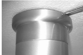
secure with set screws
