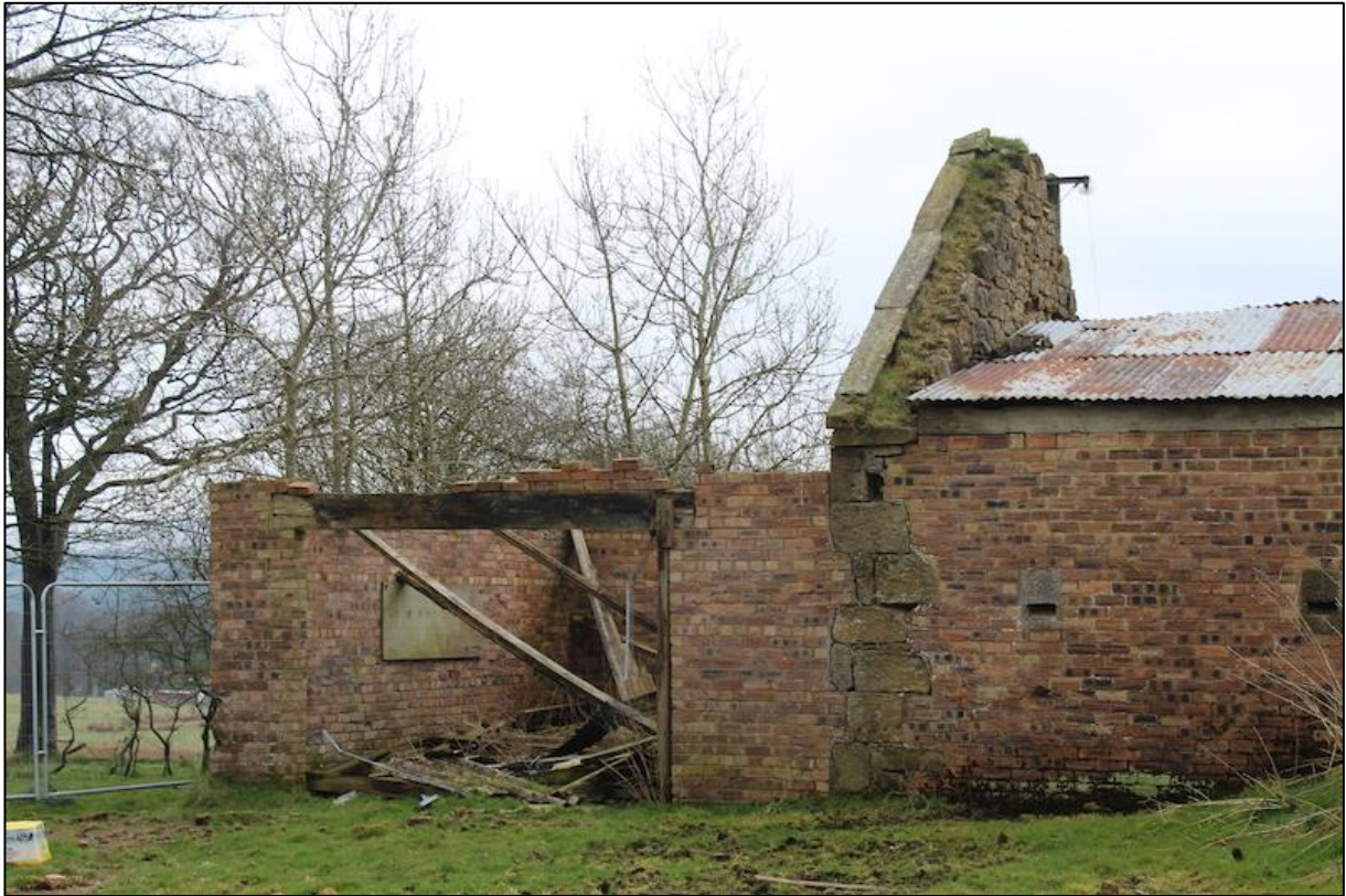
Figure 3a: Outbuildings to the S of the main house showing reuse of gable end wall.
