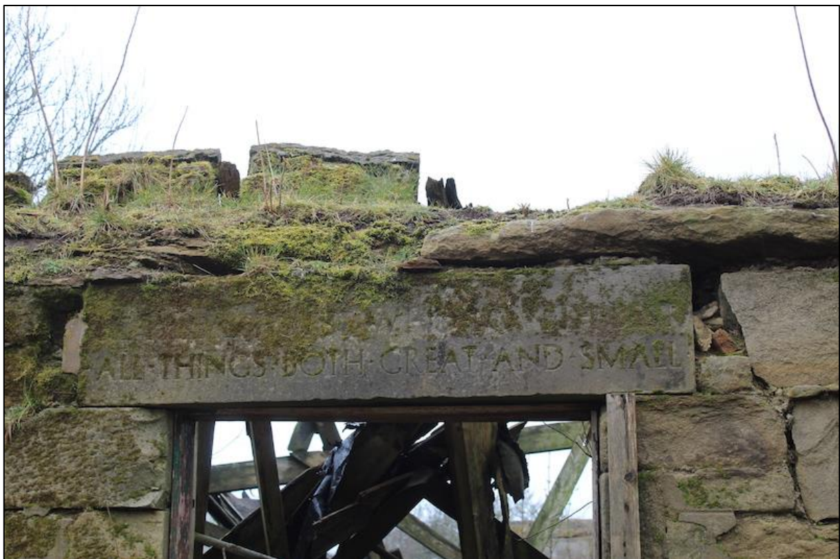
Figure 3b: Example of inscribed stones reused as lintels
