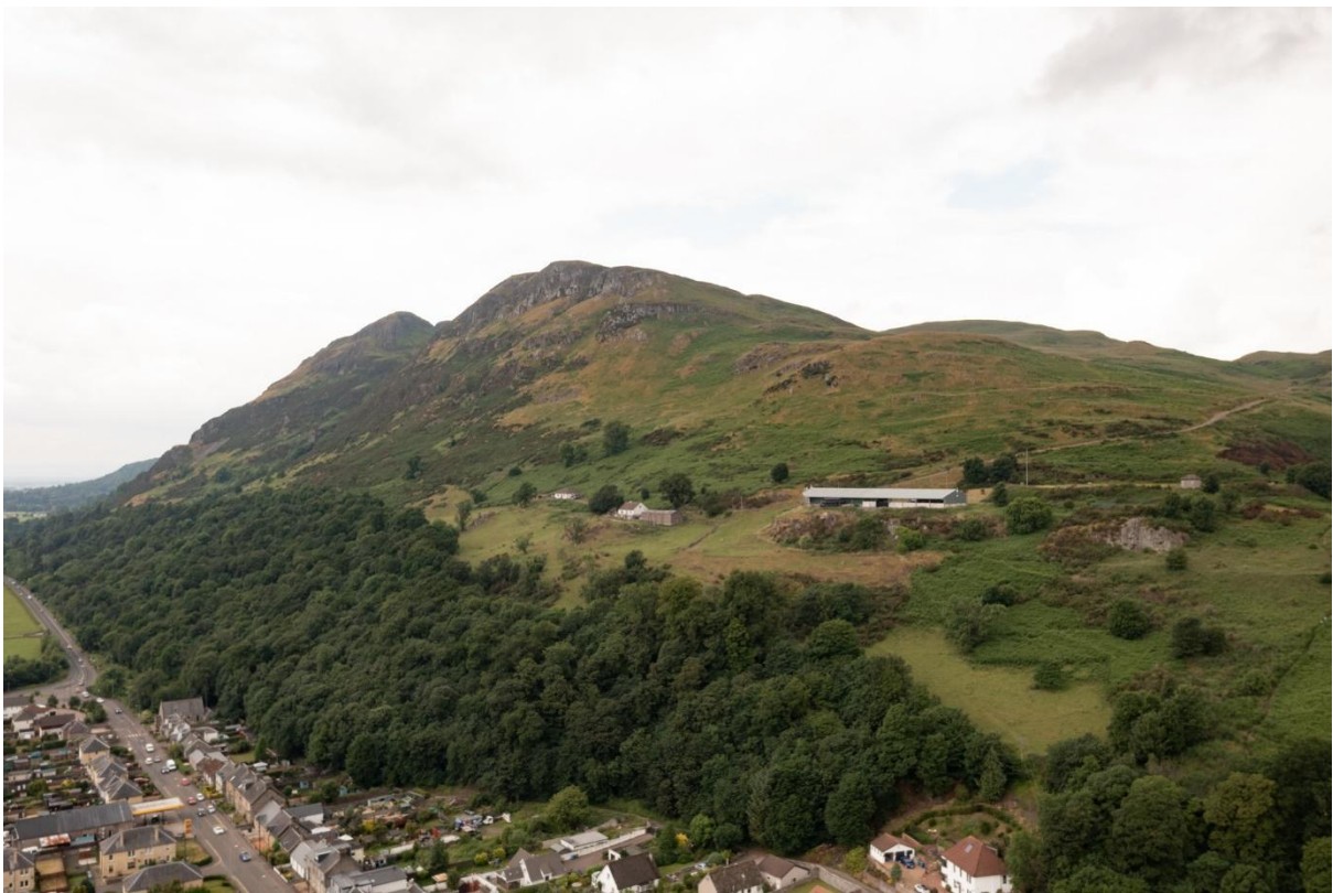
Photo 1: Dumyat Estate – looking NW – photo by FFC
