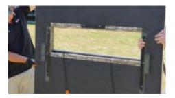
Starting with the back panel, center the panel on the end joist and hold in place. Do not attach with screws at this time.
