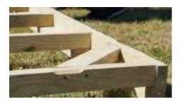
Insert corner C joists (#4) but do not attach with screws yet.
