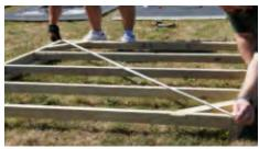
**Important:** Check for square. Rectangle should measure 98-3/4" from corner to corner for the 6x6 and 91-1/2" for the 5x6.
