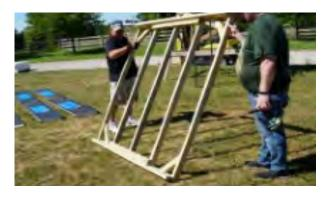
Flip floor over and screw in pre-attached bottom board K. Drive screws in fully.
