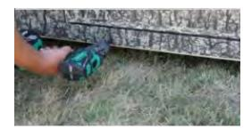
Using the 3/4" pan head screw and working 3/4" up from the bottom edge of the metal, attached screws every 4" until all walls are secured.
