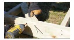
Once square is achieved, attach corner C joists with 2 screw per attachment point.
