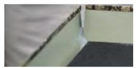
Caulk all roof interior vertical seams with clear caulk from the bottom to half way up the opening (do not smooth out with finger). The goal is to seal the opening near the SIP panel but leave the ends open so they can flex when installing the roof.
