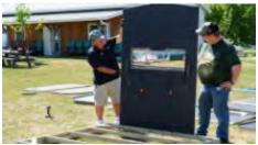
From the door position vantage point (looking at the interior back wall), add the right back corner wall by inserting the extrusion into the back panel wall. Make sure the panel is fully seated in the extrusion before proceeding.
