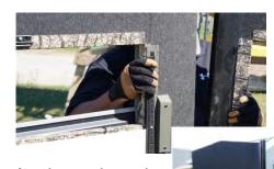
Attach extrusion and wall with 3/4" pan head screws directly opposite the preinstalled screws on the extrusion.
