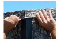
Lift the roof over the blind and gently lower onto the blind walls. *Note: Line the downward roof hem seams with the center of the extrusions.*Starting at the left back panel and working 1/2" up from the bottom edge of the roof, use 3/4" pan head screws to attach roof to each extrusion as shown on the right. Repeat in a clockwise fashion.
