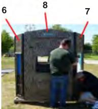
Repeat procedure above in the following order: left back corner wall, left side wall, right side wall, left front corner wall, right front corner wall and lastly the front panel with door. This completes tying all the walls together. Do not secure to the floor frame yet.
