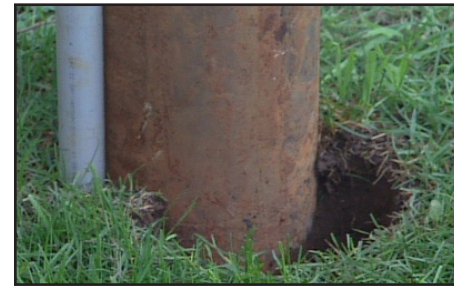
Figure 10: Drilled well with a poor or absent annular seal (Well Aware, 2017b)
