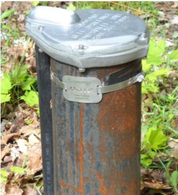
Figure 6: Drilled well (Ontario Ministry of the Environment and Climate Change, 2017b)
