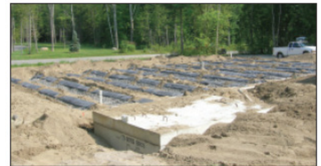
Figure 16: Septic system under construction (Government of Canada and Government of Ontario)
