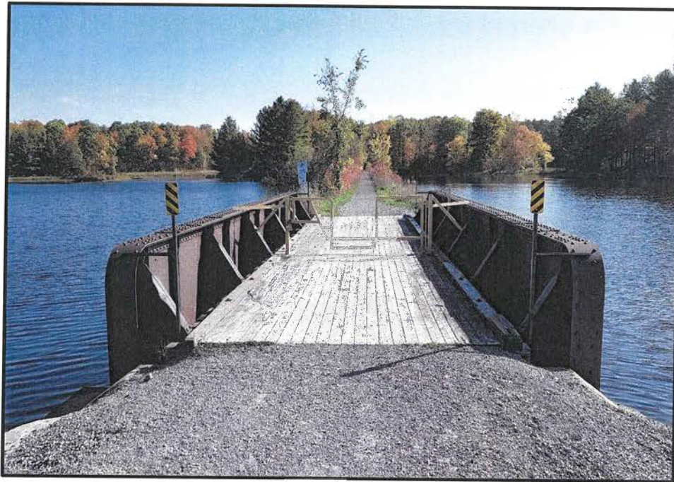
Looking East along Trail over Bridge
