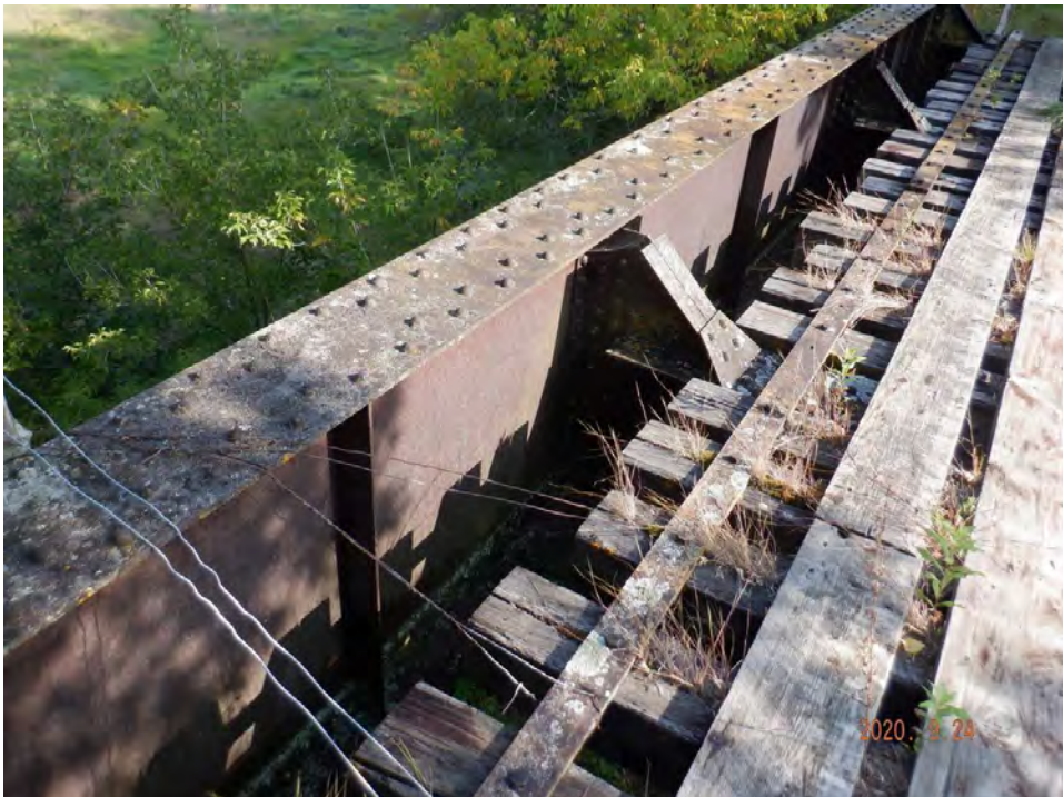
North girder detail
