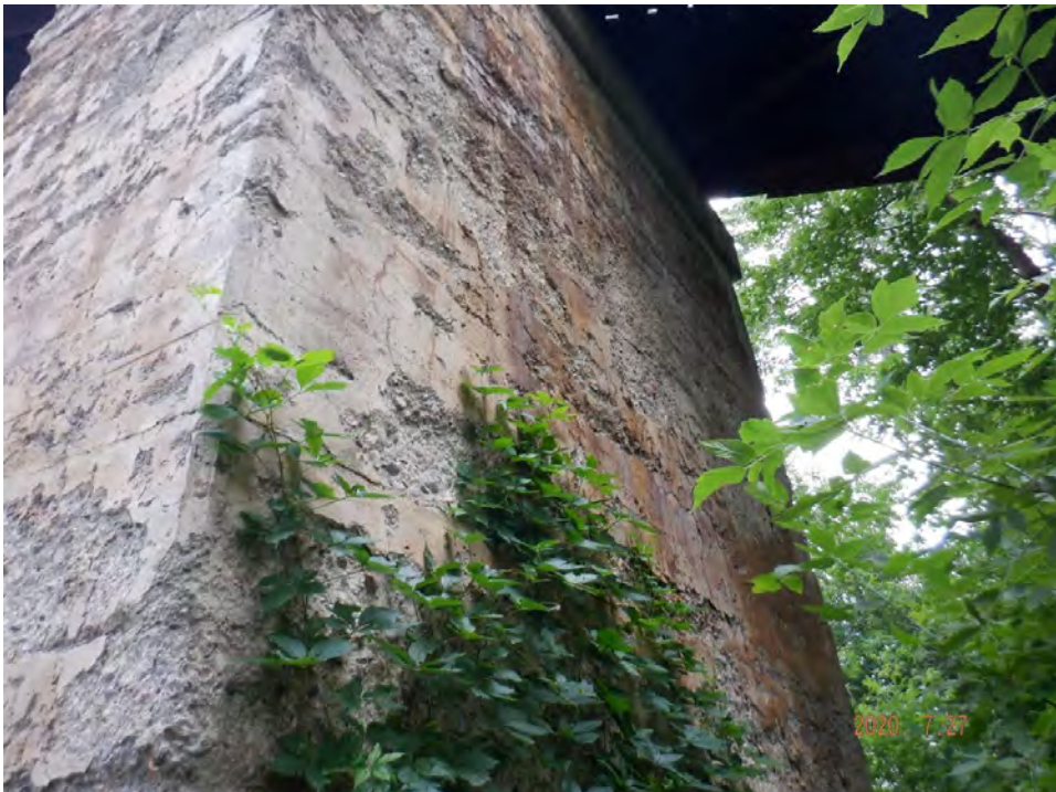
East face of pier 2
