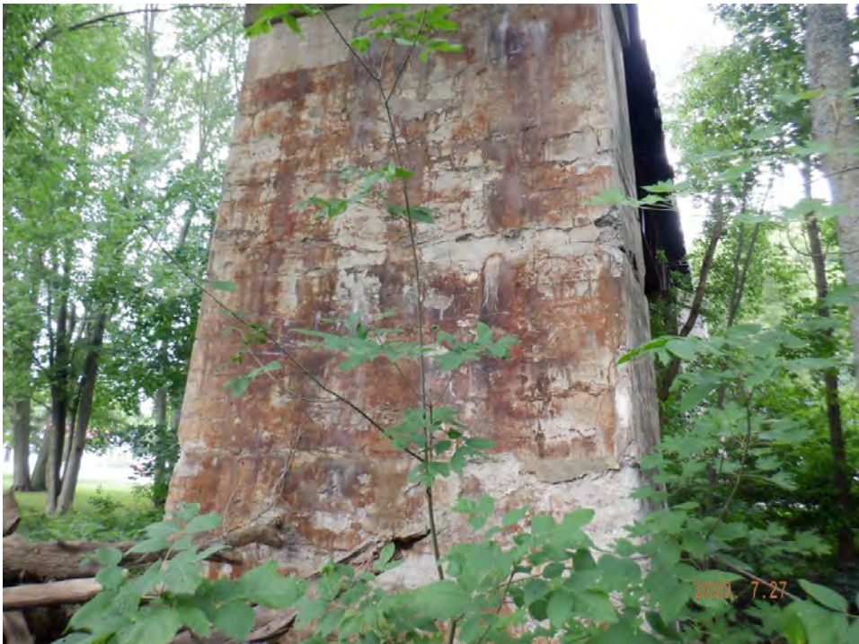
East face of pier 3
