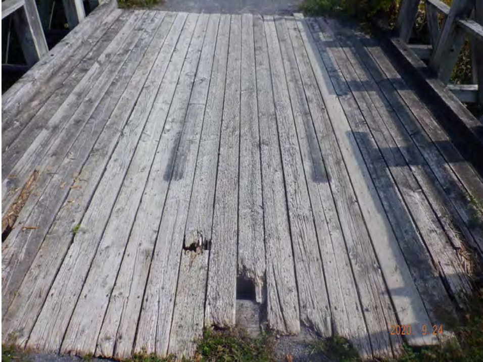
Deck wearing surface
