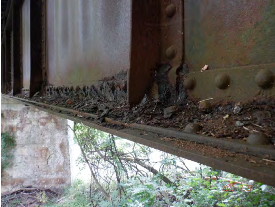
Perforated girder stiffeners in northwest
