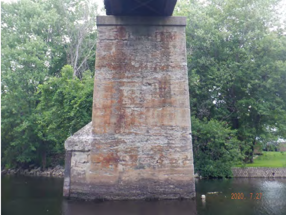
West face of pier 4
