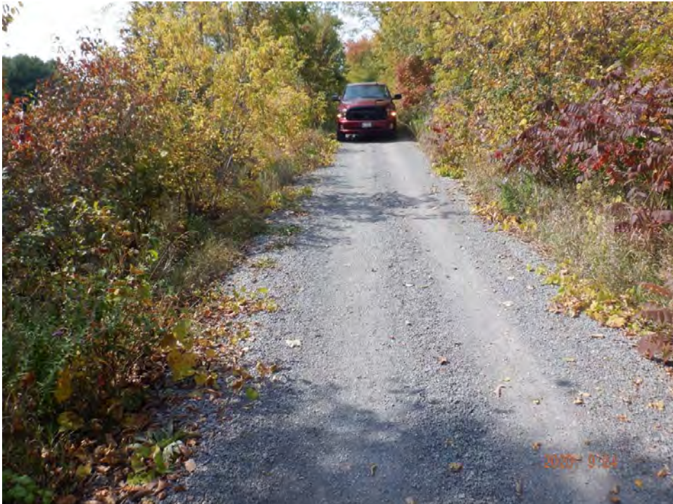
Looking west over culvert
