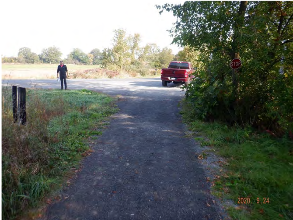
Looking north over culverts
