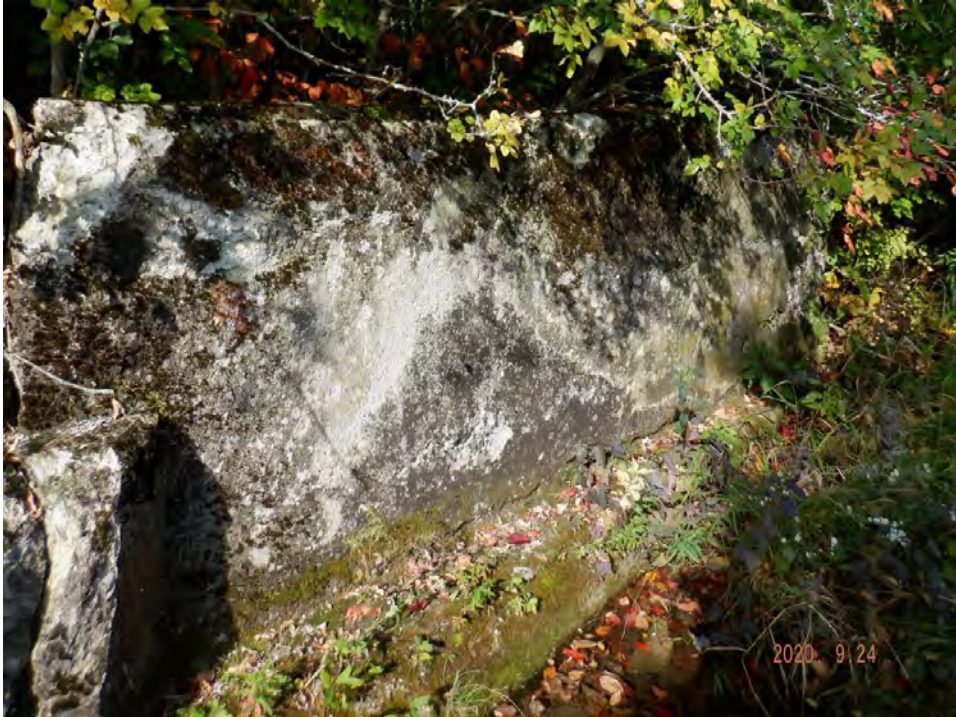
Northwest retaining wall
