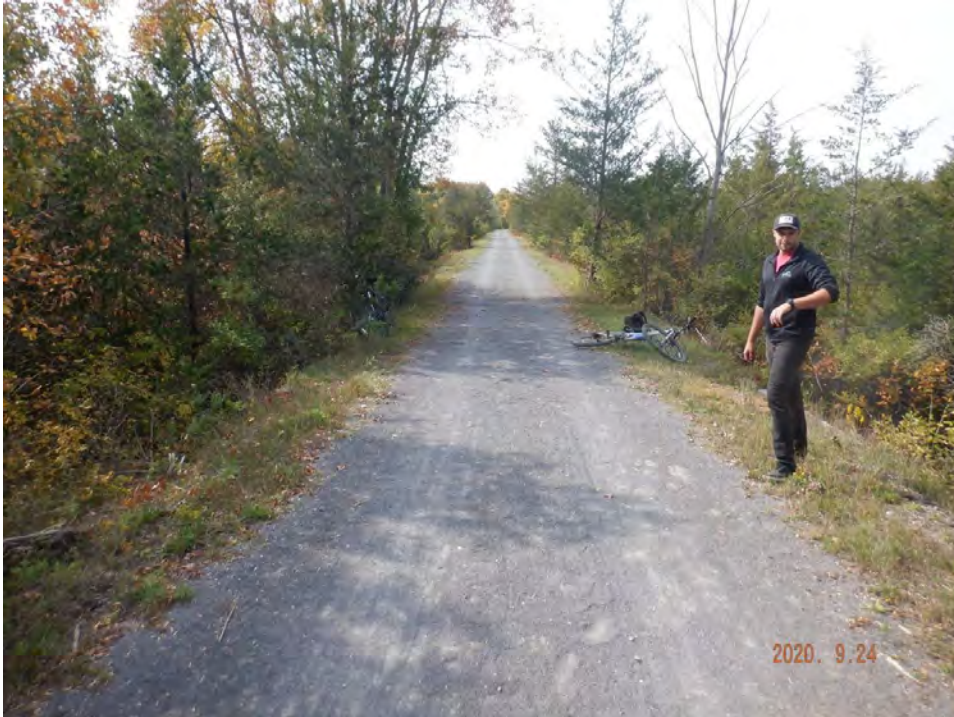
Looking west over culvert
