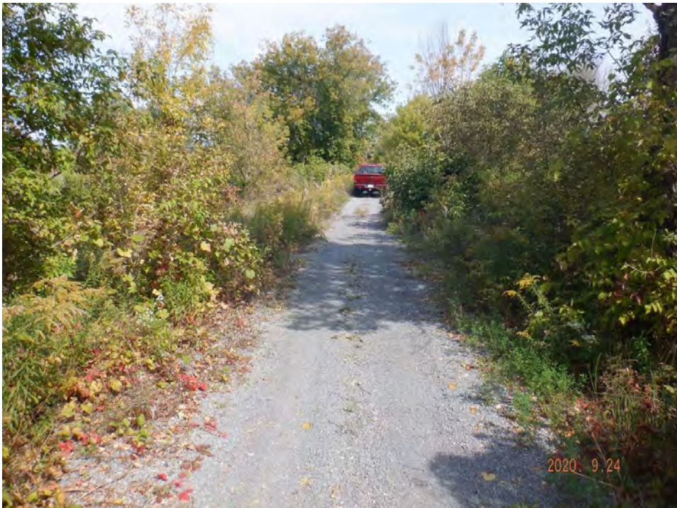
Looking west over culvert
