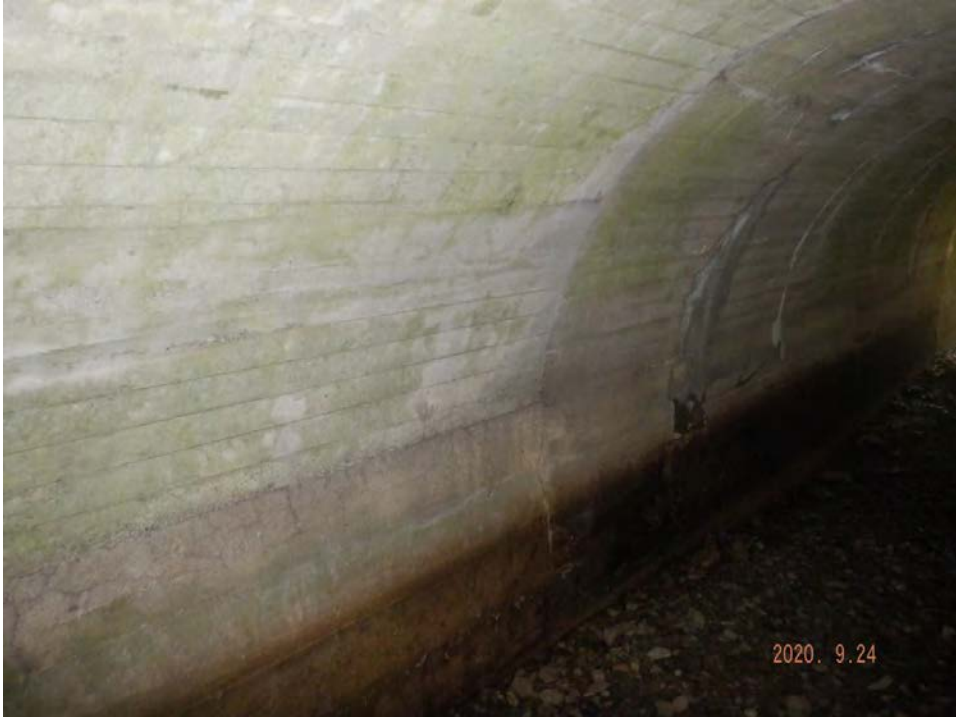
East wall (typical)
