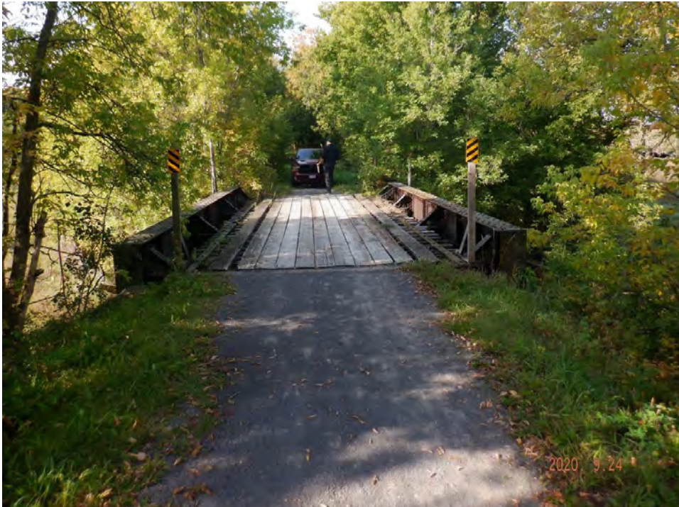
Looking west over bridge
