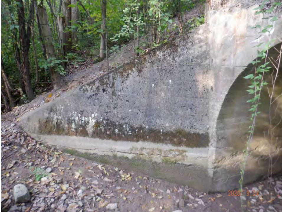
Southwest outlet wall (typical)
