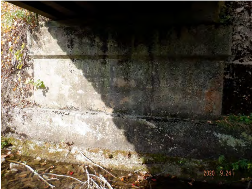
West abutment wall
