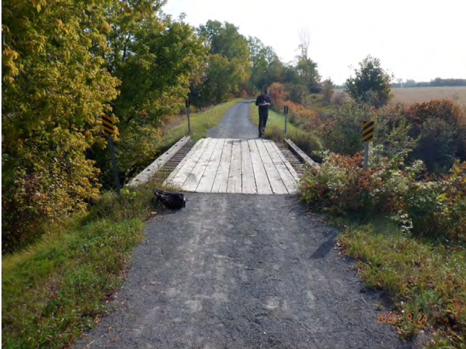
Looking east over bridge
