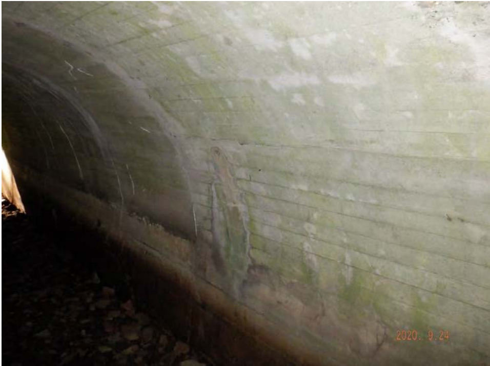
West wall (typical)
