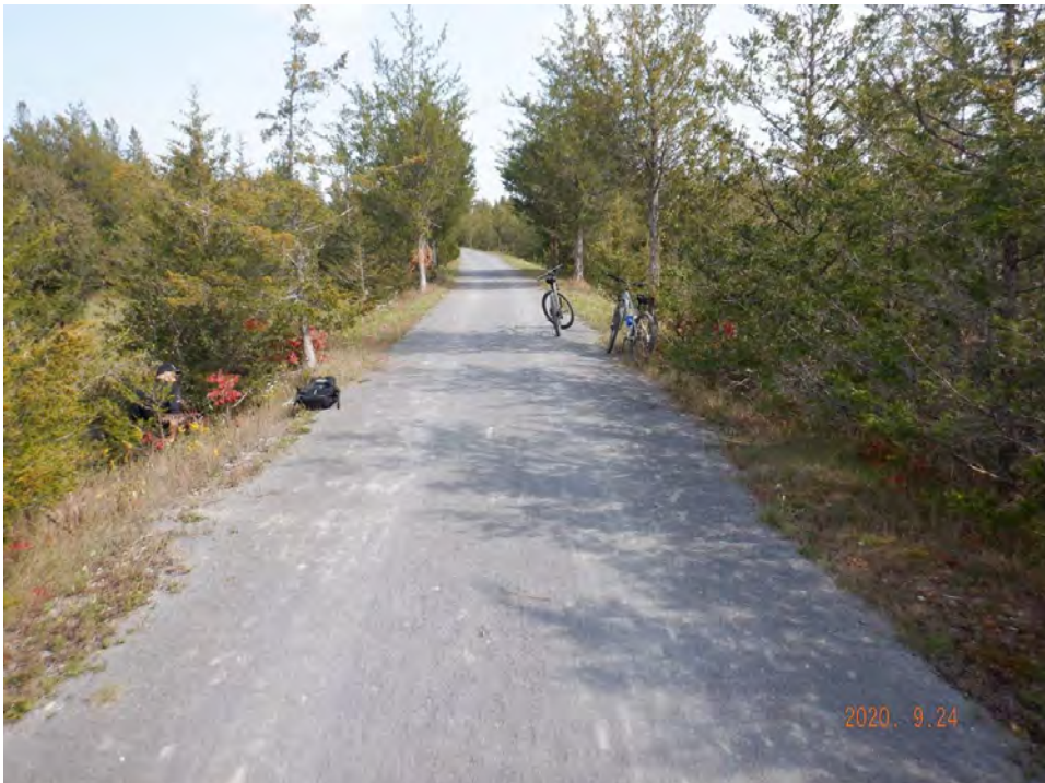
Looking east over culvert
