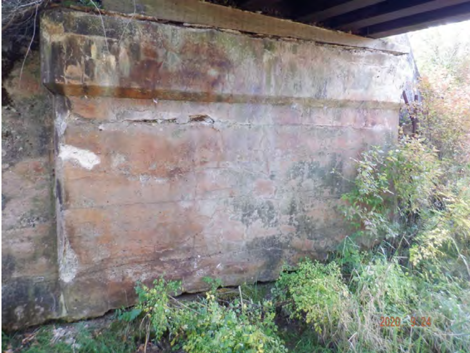
East abutment wall
