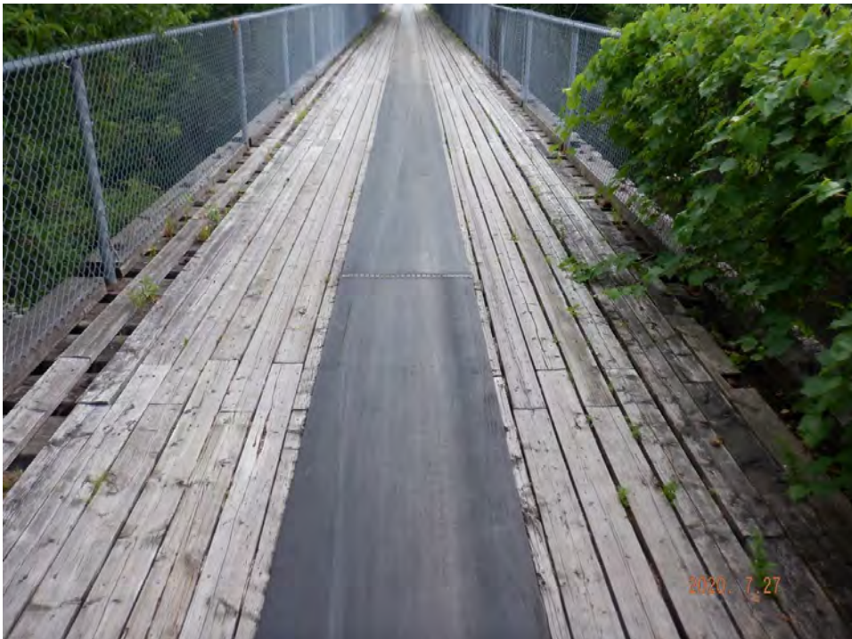
Bridge deck surface
