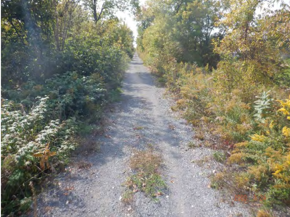
Looking east over culvert
