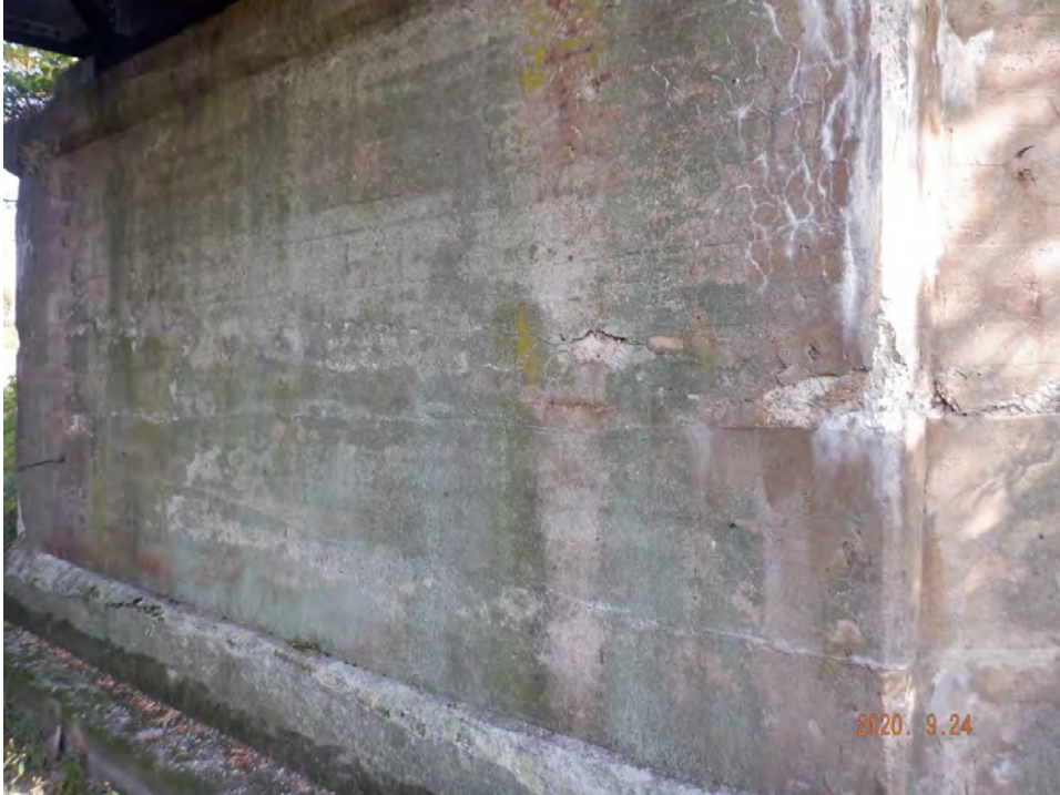
East abutment wall
