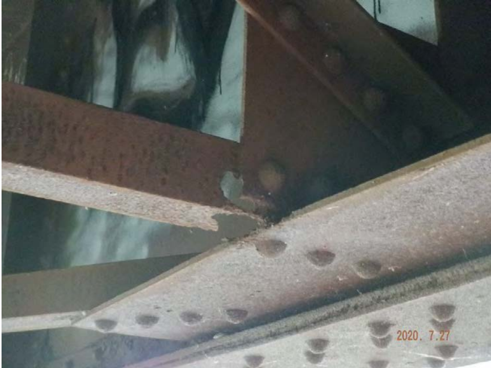
Perforated diaphragm section in northeast
