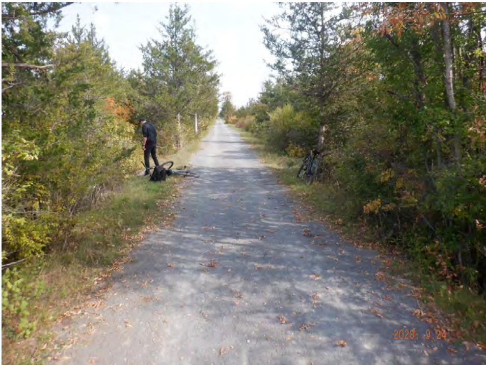
Looking east over culvert
