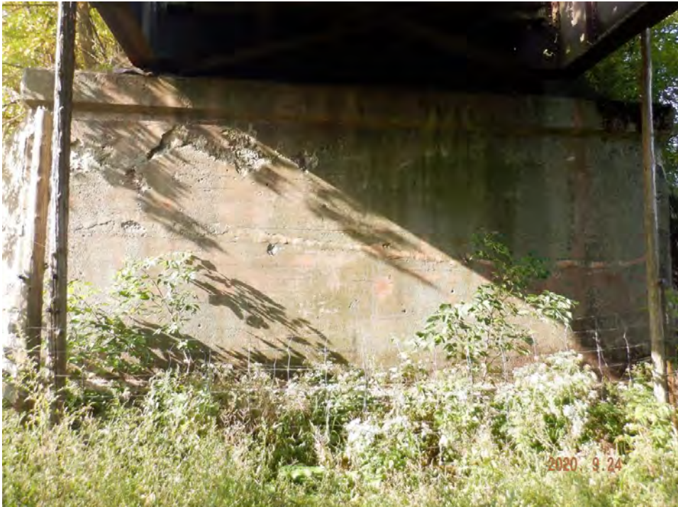
West abutment wall
