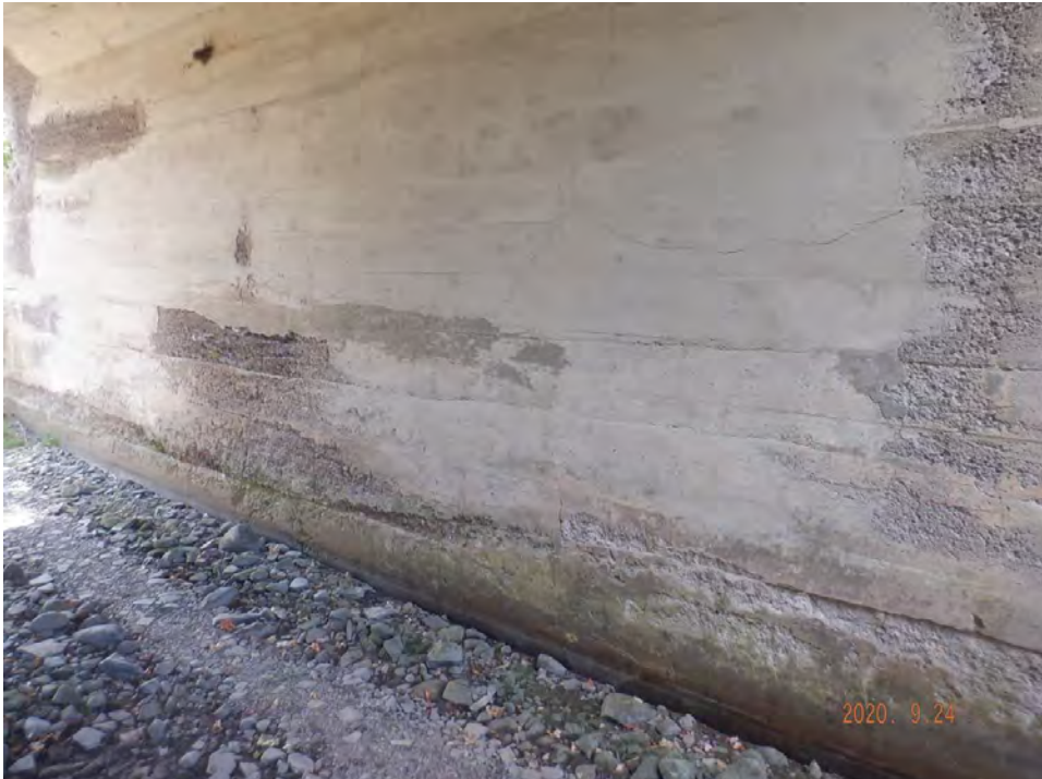
West wall (typical)
