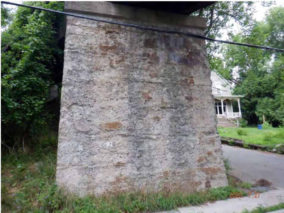
East face of pier 1
