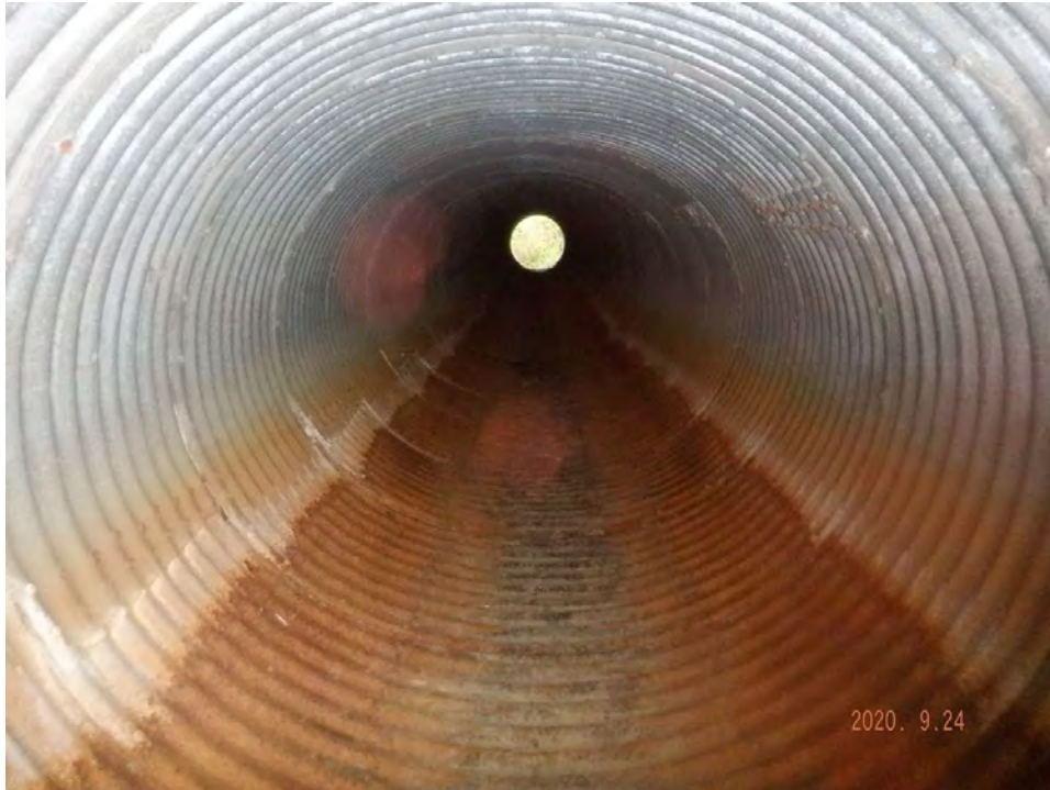
Deformation of barrel at mid length
