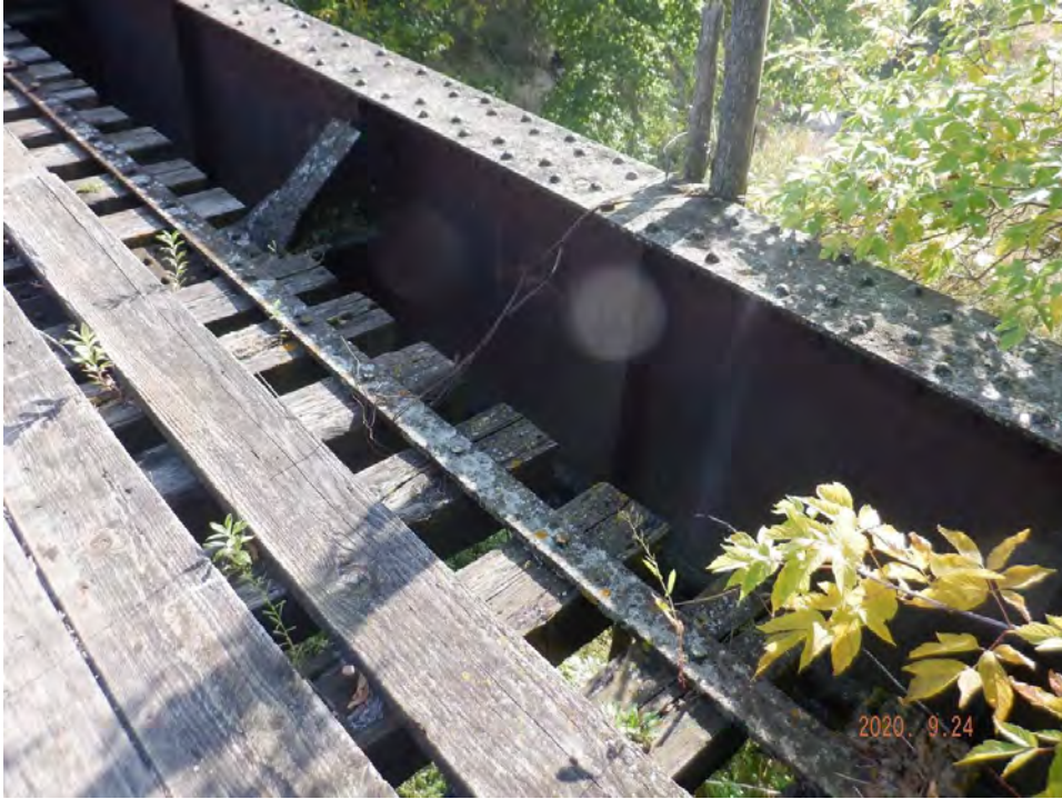
South girder detail
