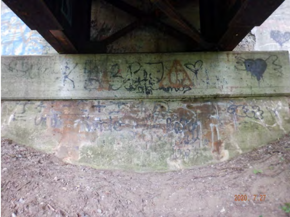
East abutment wall
