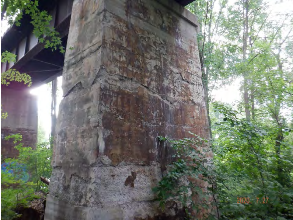
West face of pier 3
