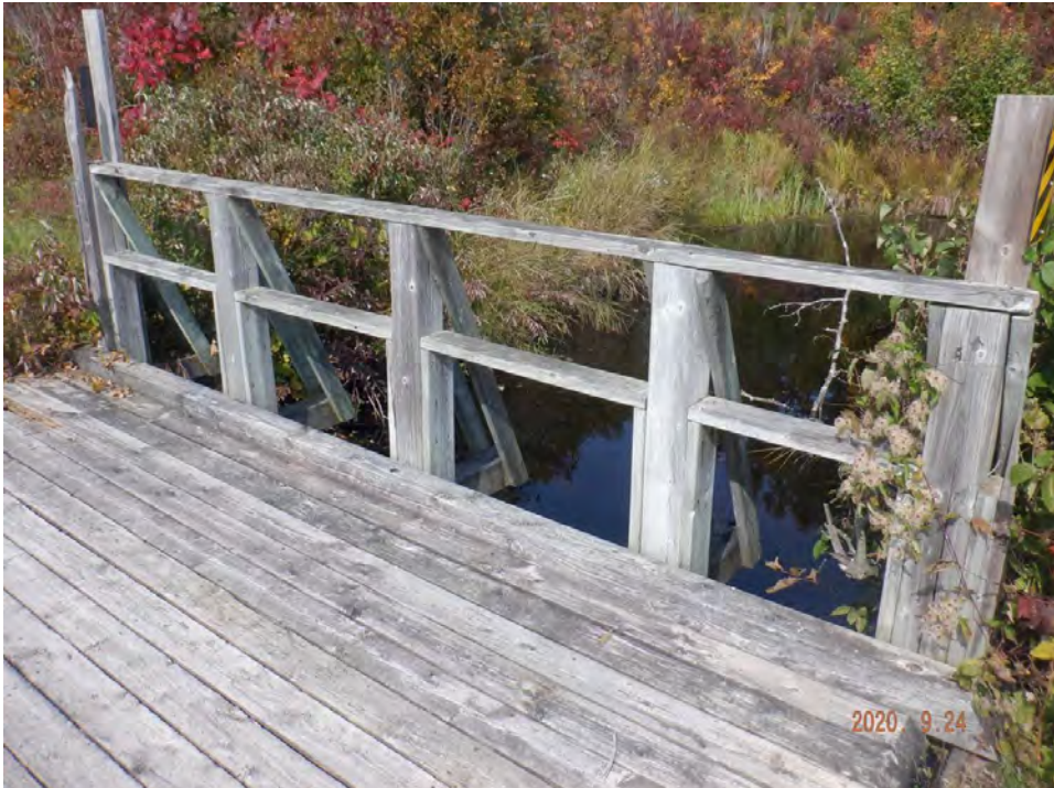
North railing system
