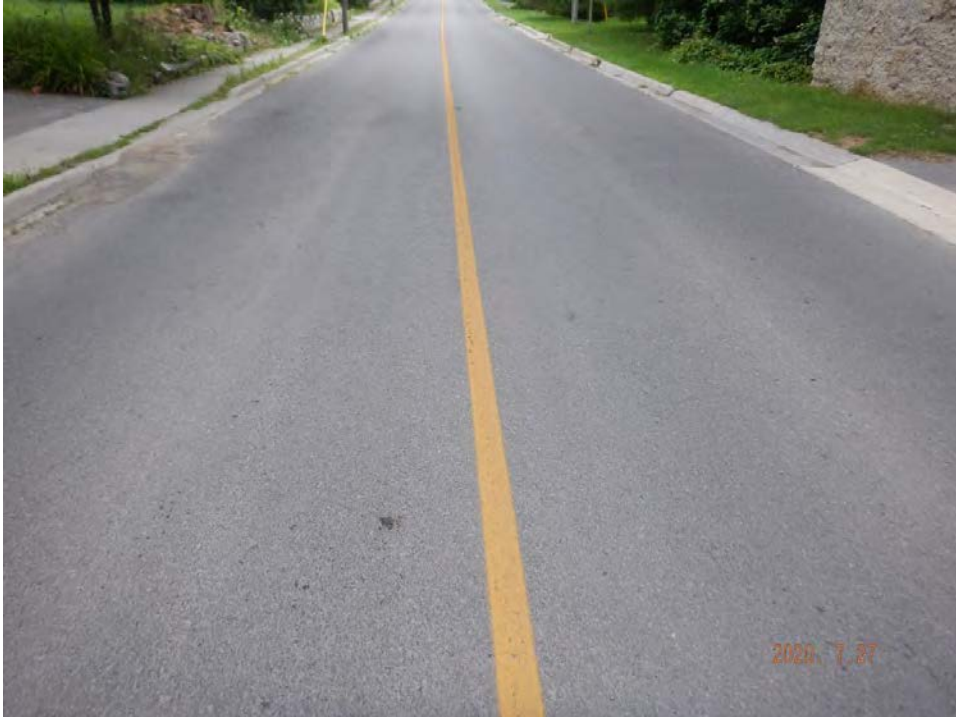
Wearing surface below bridge
