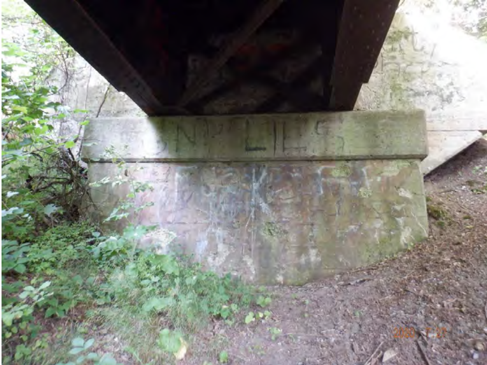
West abutment wall
