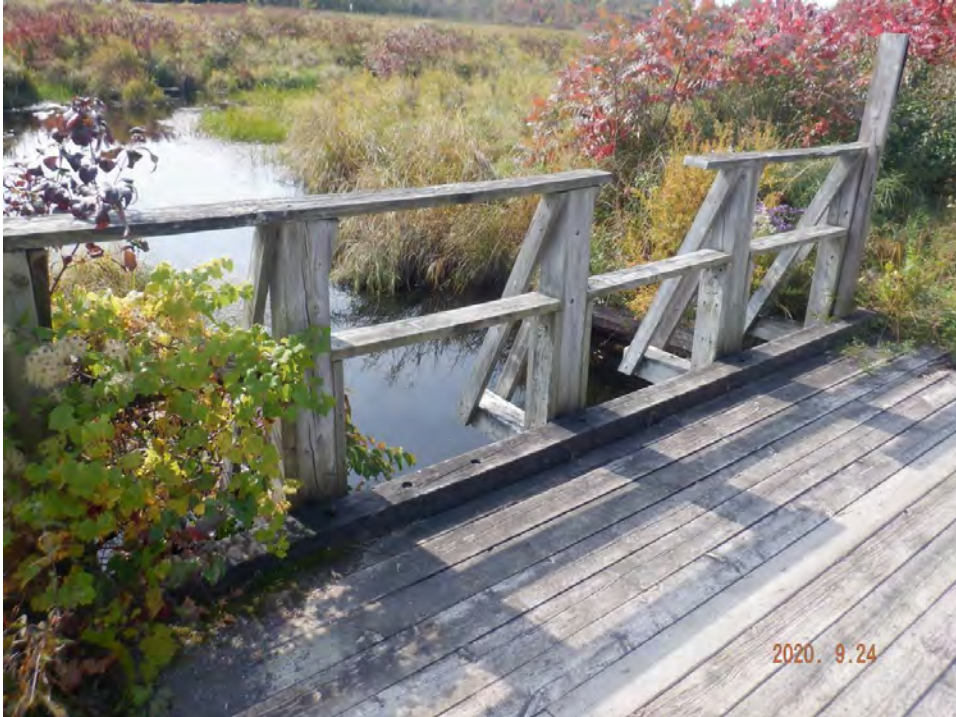
South railing system
