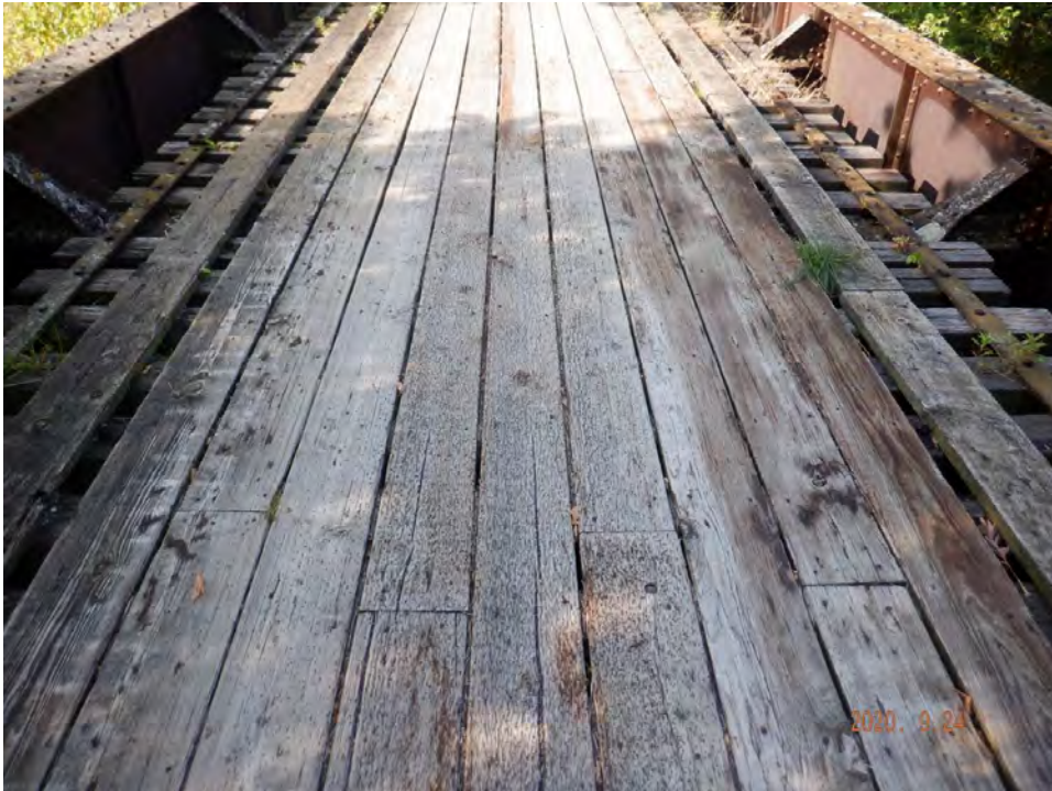
Deck wearing surface
