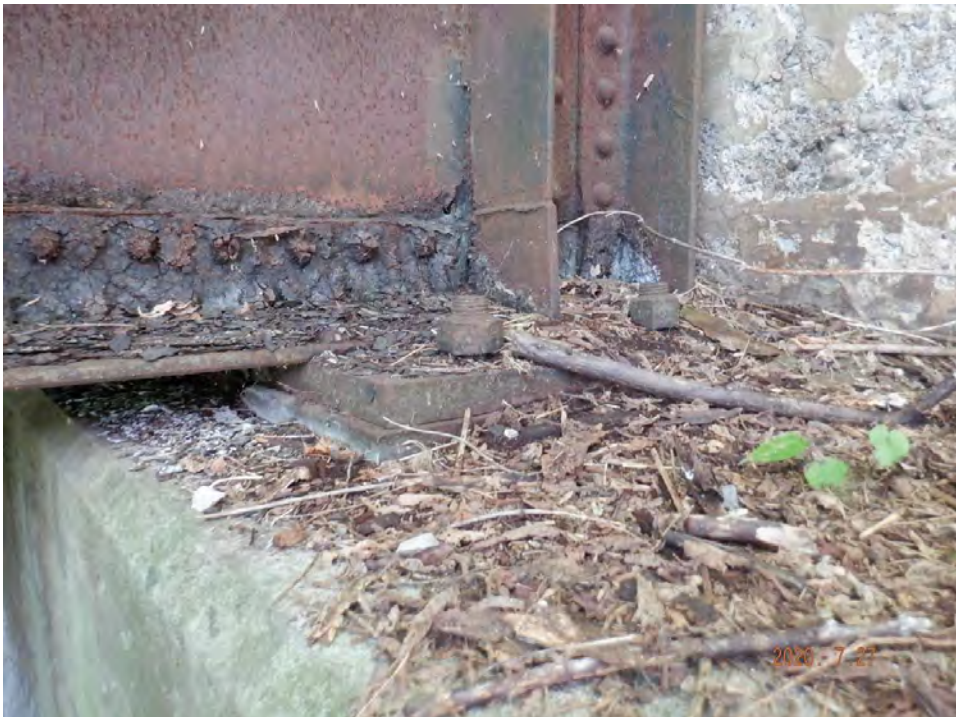
Typical abutment bearing detail
