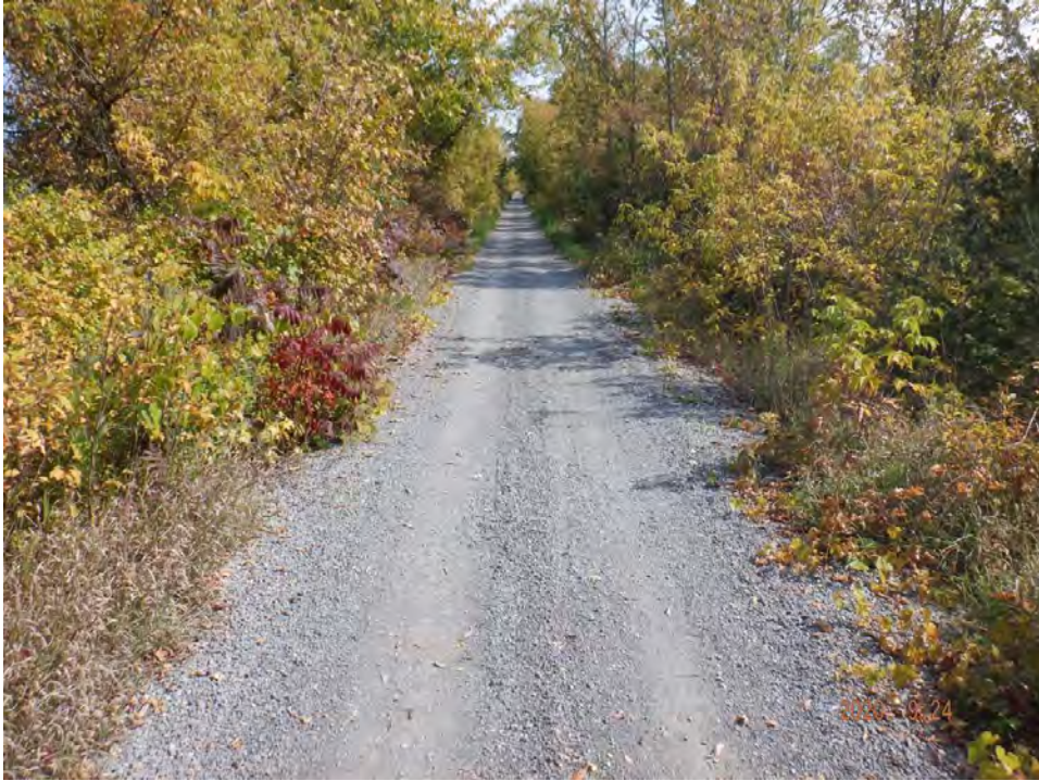
Looking east over culvert
