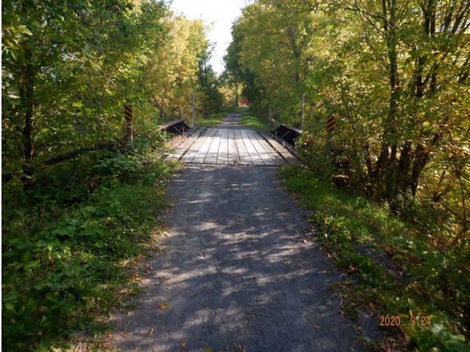
Looking east over bridge
