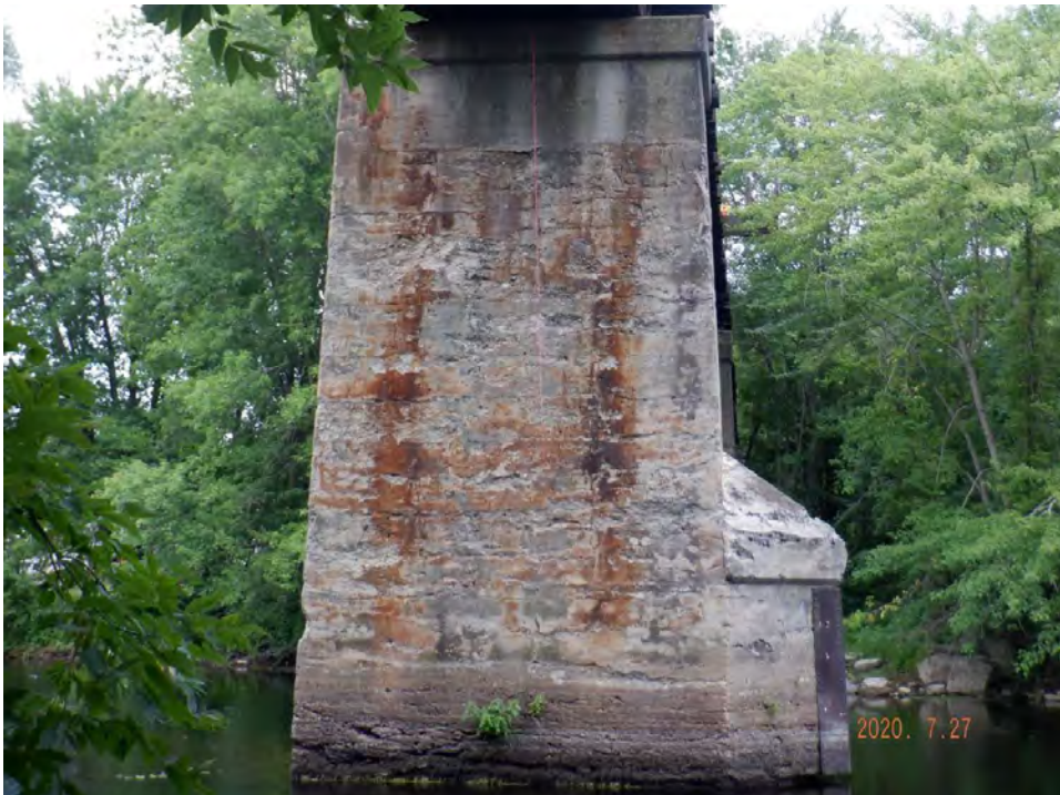
East face of pier 4
