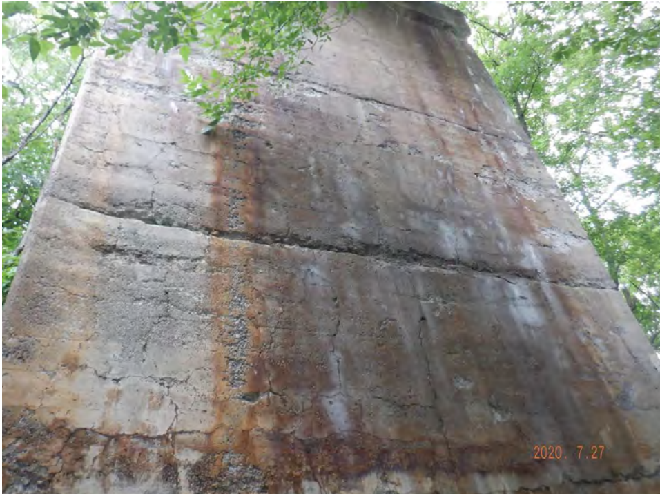
East face of pier 5
