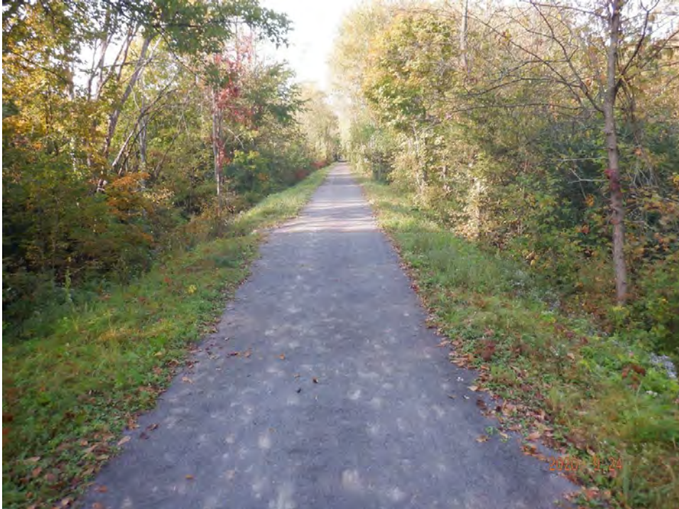
Looking east over culvert
