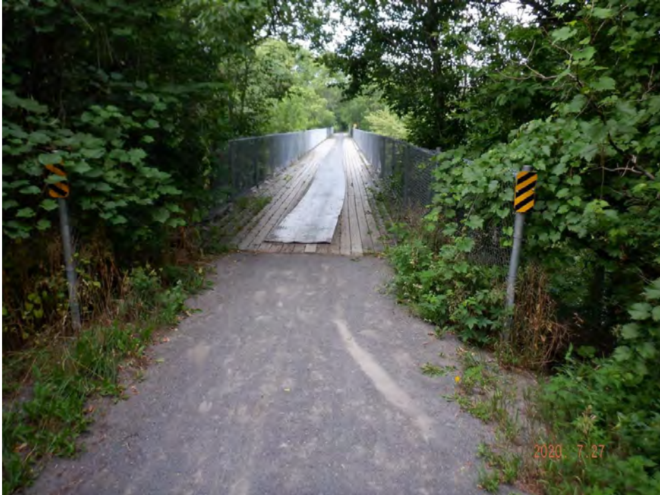
Looking west over bridge
