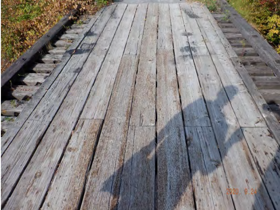
Deck wearing surface
