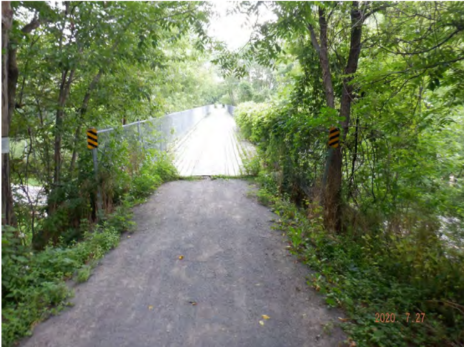
Looking east over bridge
