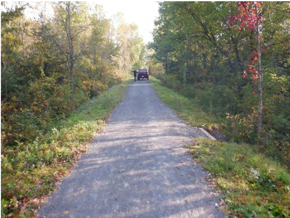
Looking west over culvert
