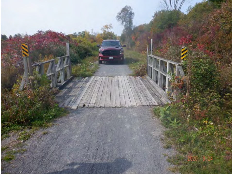
Looking wst over bridge
