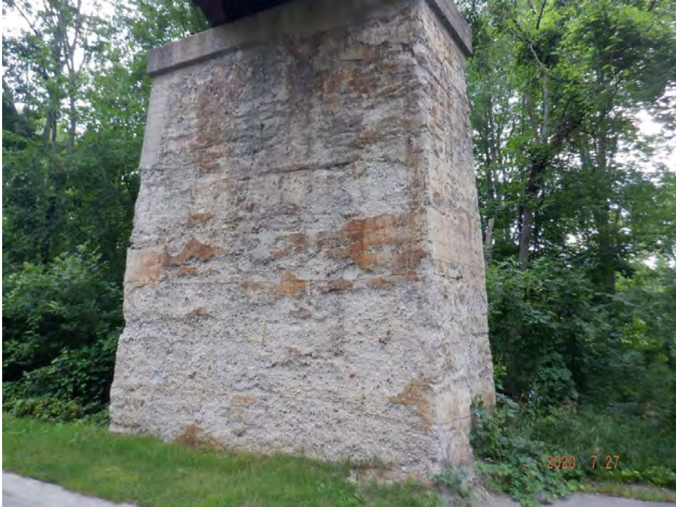
West face of pier 2
