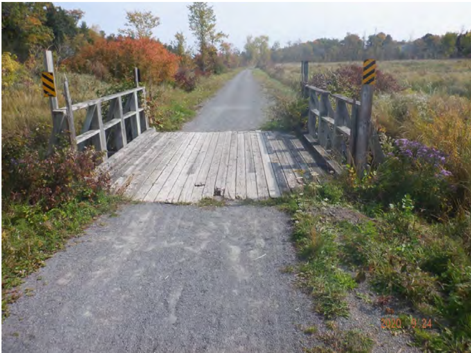
Looking east over bridge
