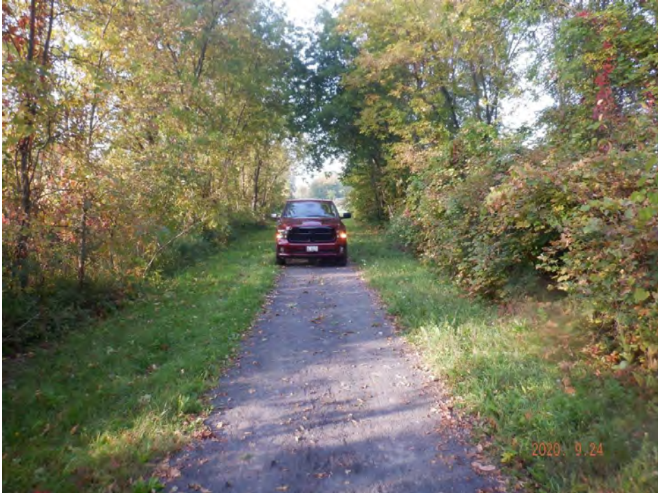
Looking West over culvert
