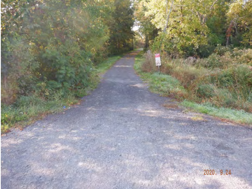
Looking south over culverts
