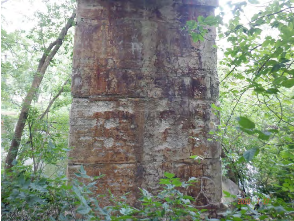
West face of pier 5
