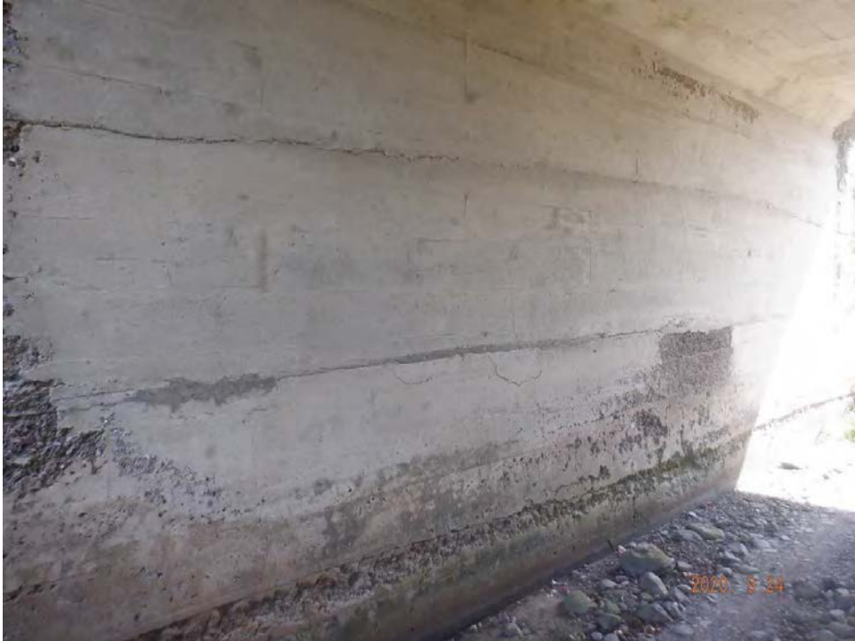
East wall (typical)
