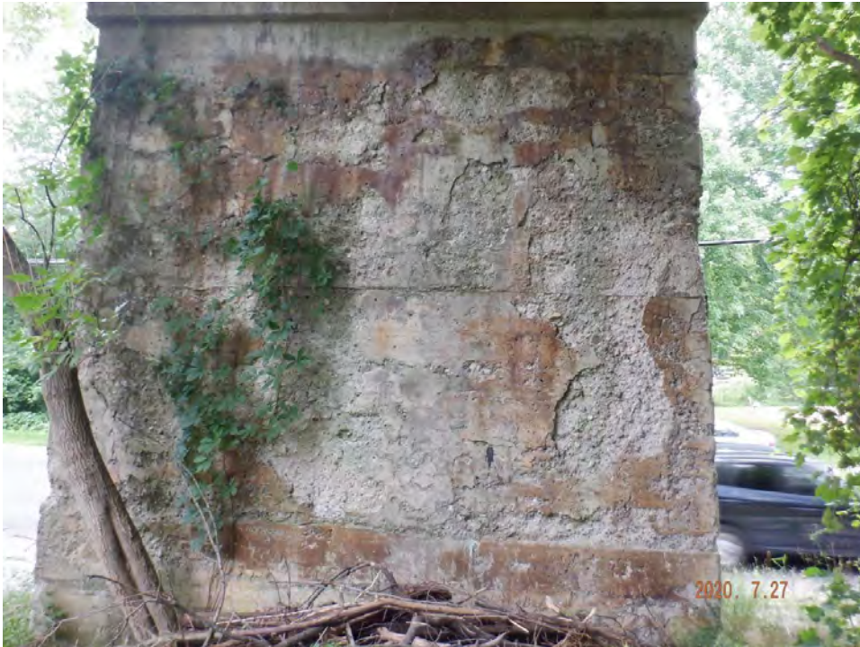
West face of pier 1 (west to east)
