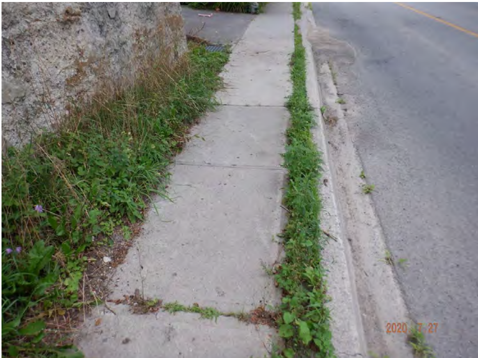
Sidewalk below bridge
