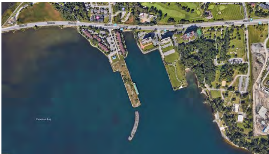
Figure 30 Elevator Bay, Kingston
