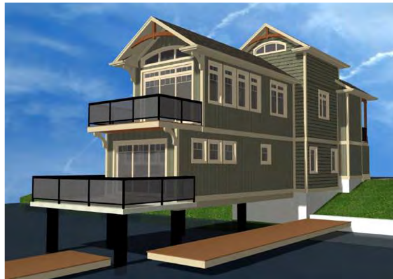
Figure 29 Piled over-water residential development.
