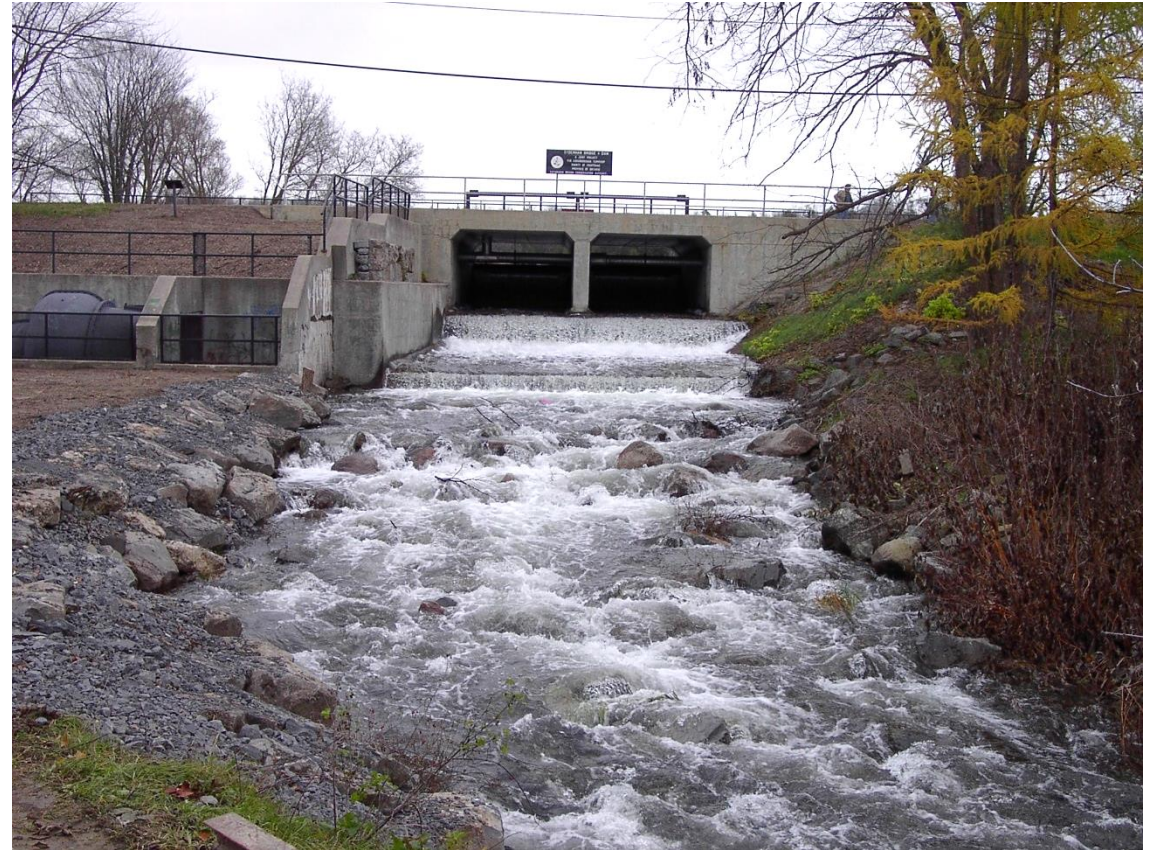
Sydenham Water Control Structure
