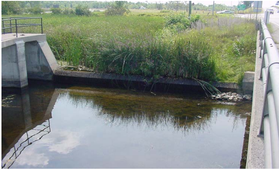
PHOTO WIL-13: SOUTH SIDE WEIR
