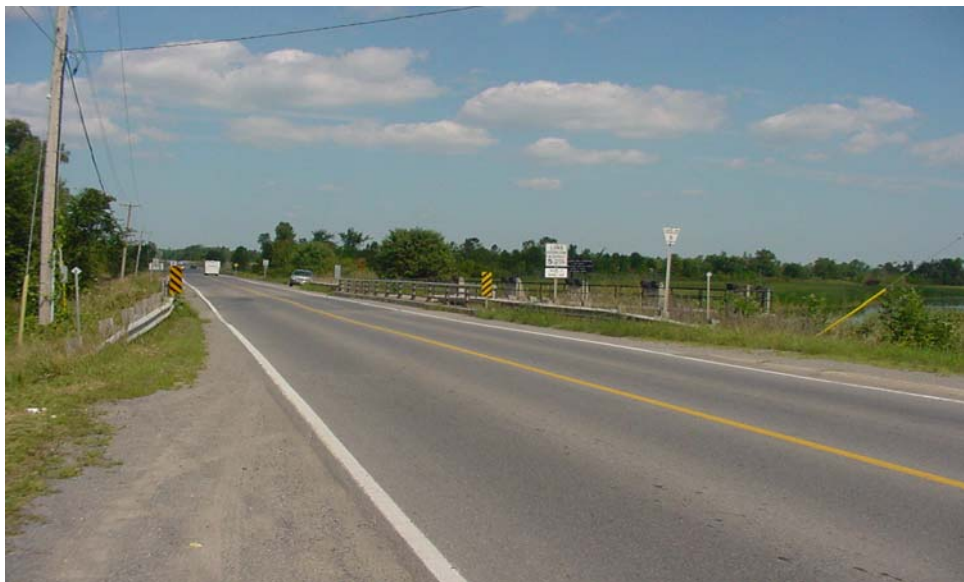
PHOTO WIL-02: WILTON ROAD, BRIDGE IN CENTRE (VIEW NORTH)
