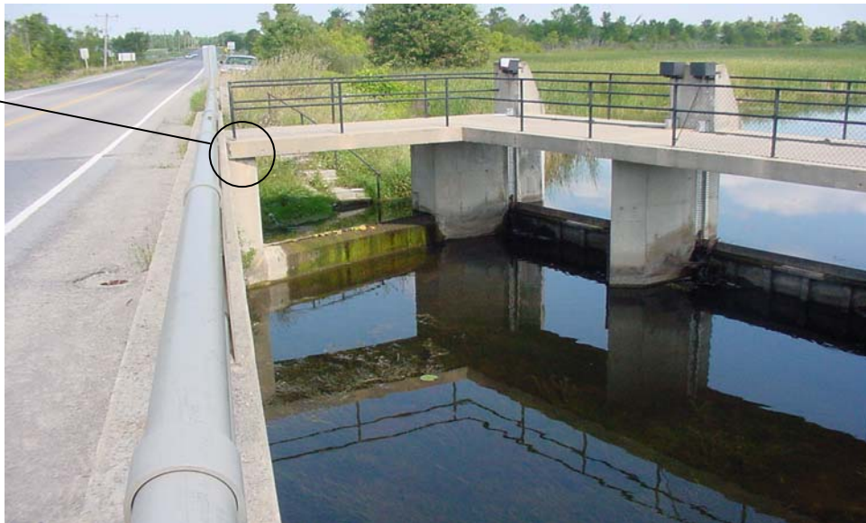
PHOTO WIL-12: NORTH SIDE WEIR
