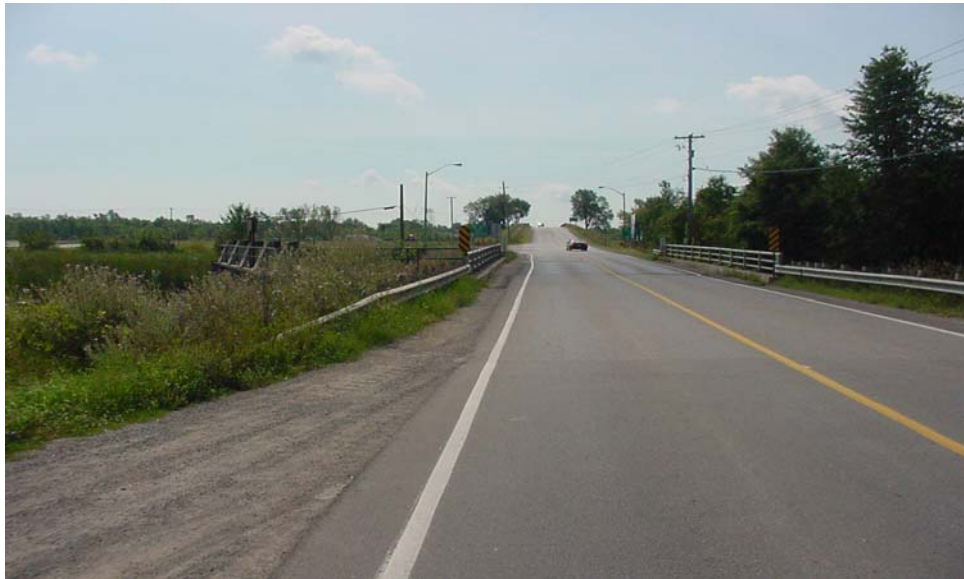
PHOTO WIL-01: WILTON ROAD, DAM ON LEFT (VIEW SOUTH)
