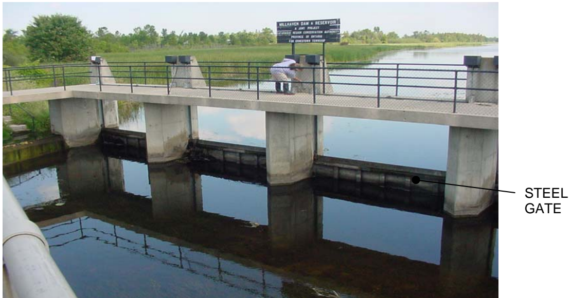
PHOTO WIL-10: STEEL GATES IN BAYS
