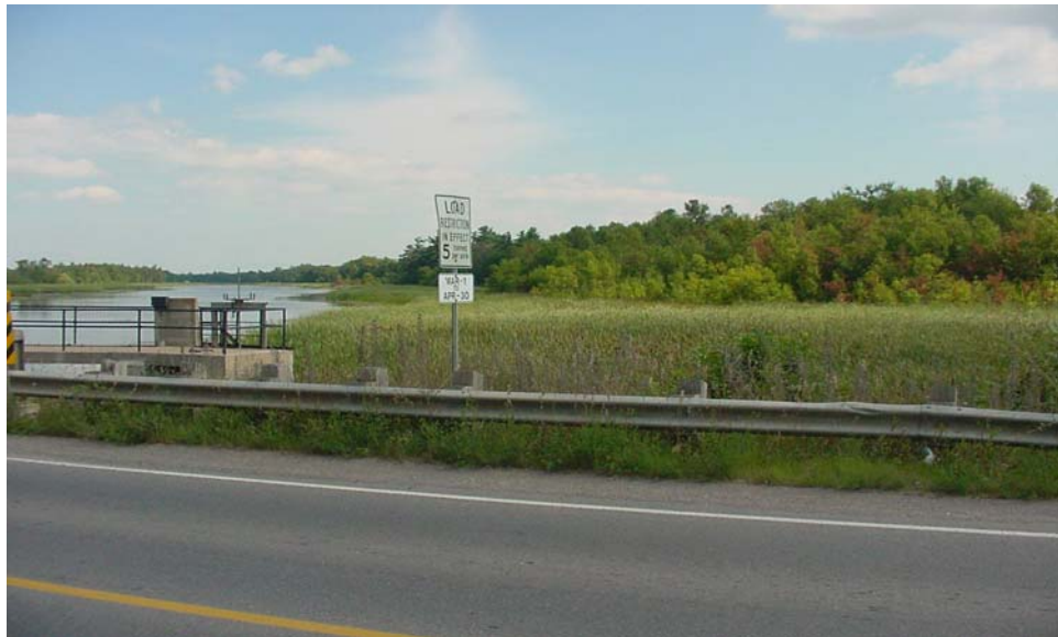
PHOTO WIL-04: SOUTH SHORELINE (UPSTREAM)
