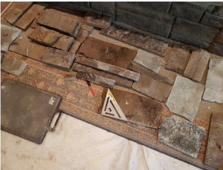
Below: Example of cut stone.
