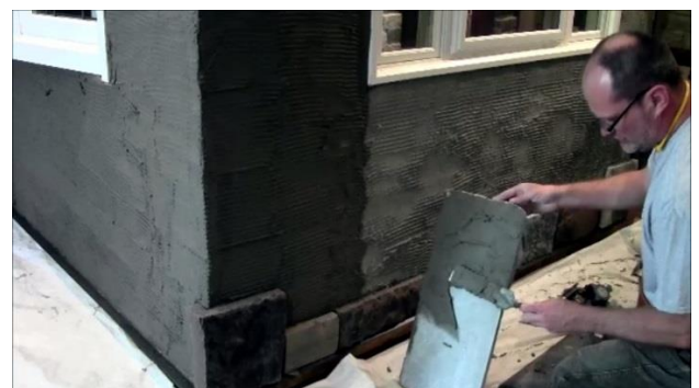
Above and below, examples of applying mortar directly to back of stone. Also referred to as "buttering" back of stone.
