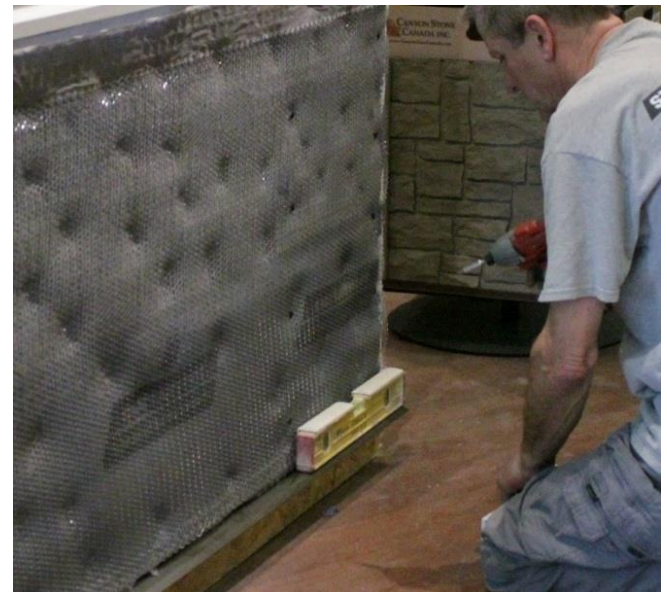
Metal lath being fastened to wall
