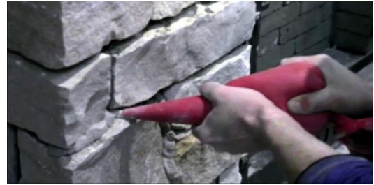
Above: Example of joint grouting.
