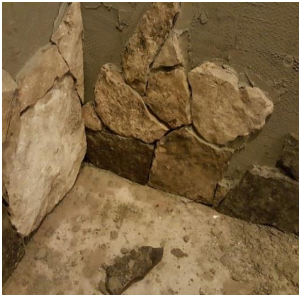
Below: Example of passing stone at inside corners.
