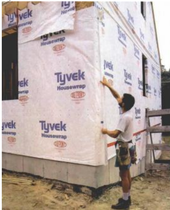
WRB being installed to structure.
