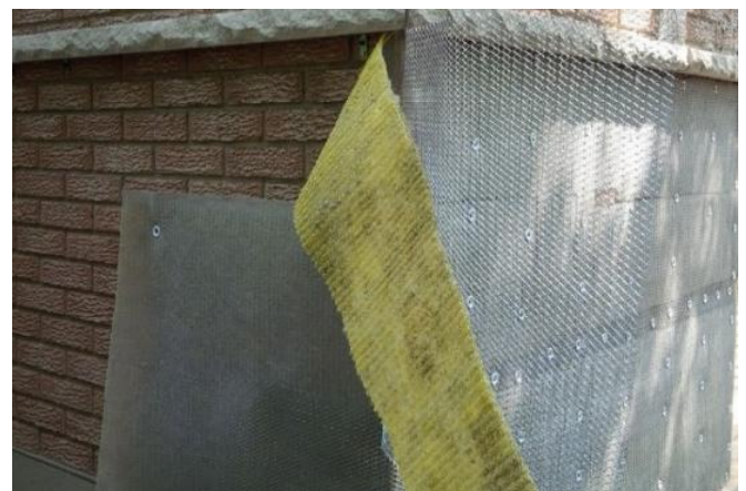
Metal lath attached to exterior brick veneer.
