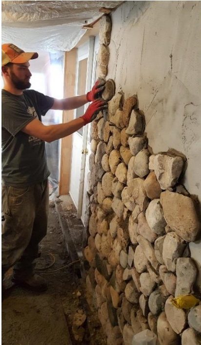
Above: Placing stone on prepared wall.
