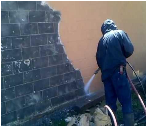
Sandblasting CMU wall to remove non-cementitious material.
