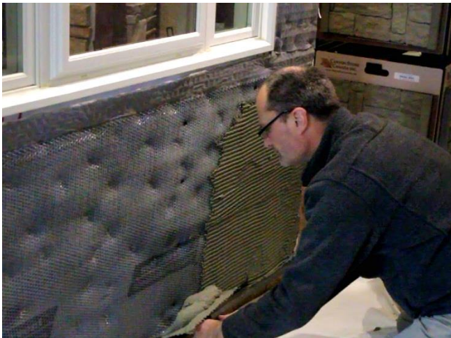
Scratch coat being applied to metal lath.
