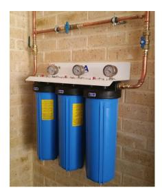
The Big Blue Systems are UV resistant however where possible it is best for the longevity of the system to install the unit undercover, or construct a simple cover for the system to shield it from direct sunlight and weather extremes such as rain, storms and frost.
