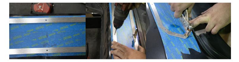
4) Once the back plate is aligned, trace out the interior and all holes. Start the cut in the corners with the dremel equipped with a cutoff wheel.(CUT OUTSIDE LINES BUT NOT TOO FAR, WATCH OUT FOR HOLE MARKINGS)
