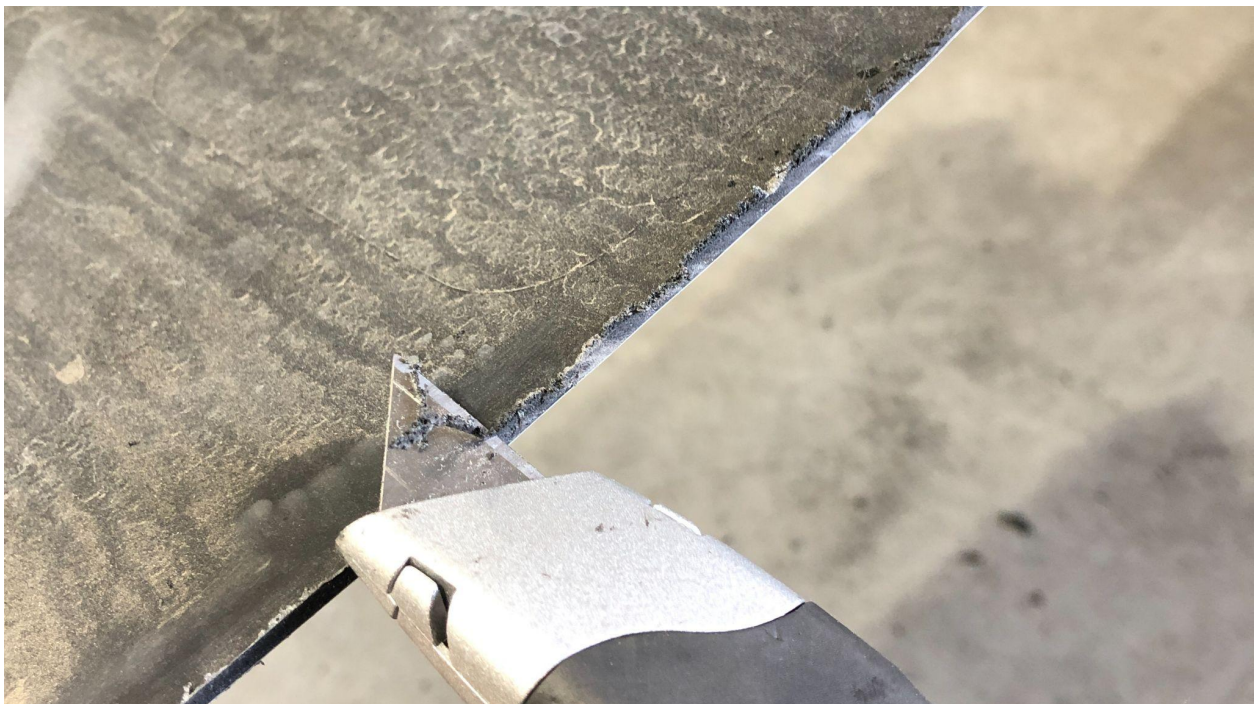
6) Clean up edge with razor knife or sanding block
