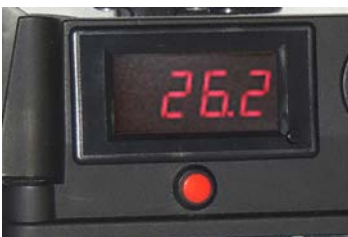
Figure 3 Amp meter showing the charge rate from an outlet socket
