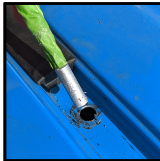
Be careful not to drill too deep, use a step bit or drill stop. A magnet can be used to clean up any excess shavings
