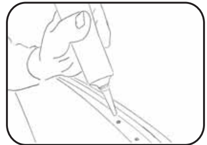
Silicone holes in roof.
