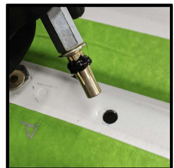
Place a thin bead of silicone around the plusnut then insert it into the roof
