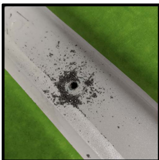
In the locations where the rear channel trim bolts were expand the holes to 3/8"
