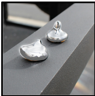
Apply a generous amount of silicon to the holes as shown above
