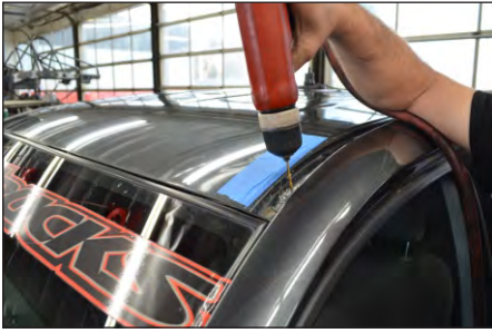
STEP 7 - Drill holes with pilot drill bit, then work up to 3/8" hole.
