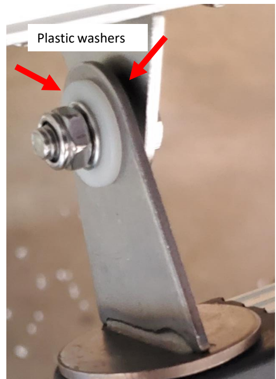
Ladder to ladder bracket attachment
