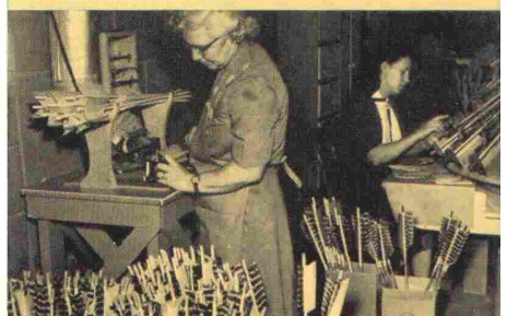
With glowing wire, feathers are trimmed to final shape.
