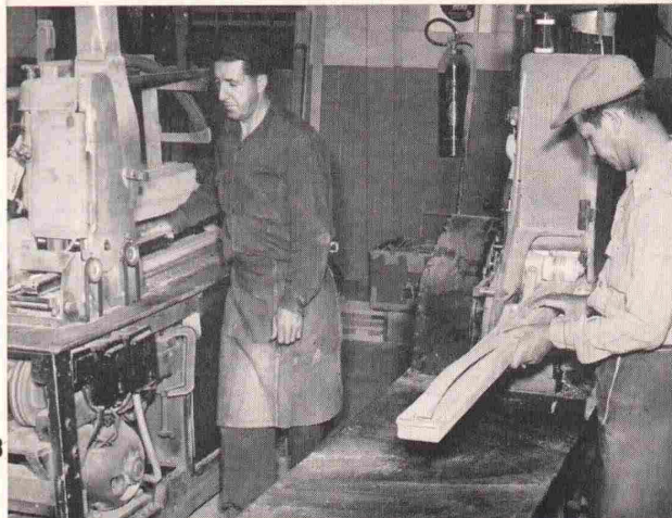
Precision sanding each piece of bow core stock and Fiberglas to exact size and uniform thickness. Pieces must be accurate and parallel to .001 in., insuring uniformly accurate shooting.
