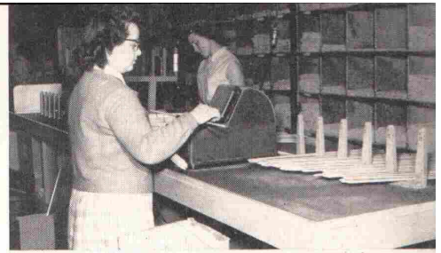
Selecting, weighing and classifying arrow shafts with aid of shadowgraph scale.
