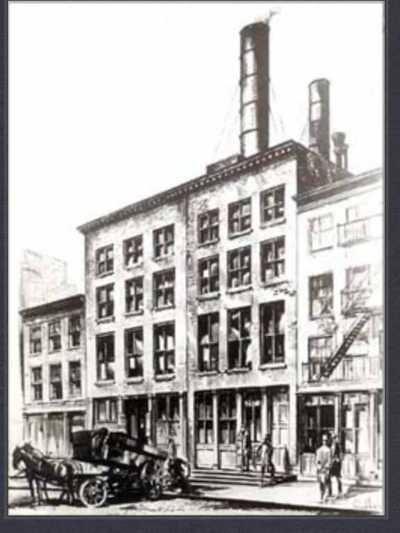
The term 'DE' may be relatively new, but the concept is as old as commercial electricity. The very first power plant in the world, in New York City in 1882, provided both electricity and useful heat to the neighboring buildings.
