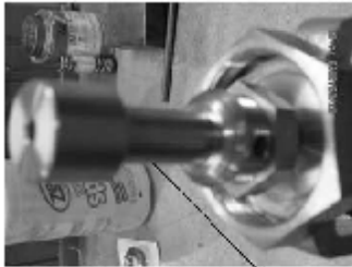
Inspect main valve.
