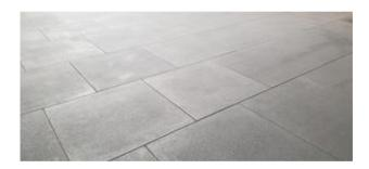
When installing the mats, bear in mind that you can compress them with a variance of up to **10mm** easily. Depending on the thickness of the mat, this variance can be even more.
