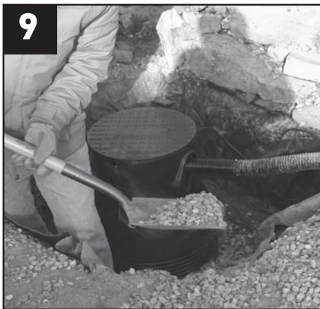
Fill the basin part way with 3/4" round gravel or small cobble by hand. Washing rocks and gravel prior to installation will reduce dust and debris that can cause cloudy water at startup.
