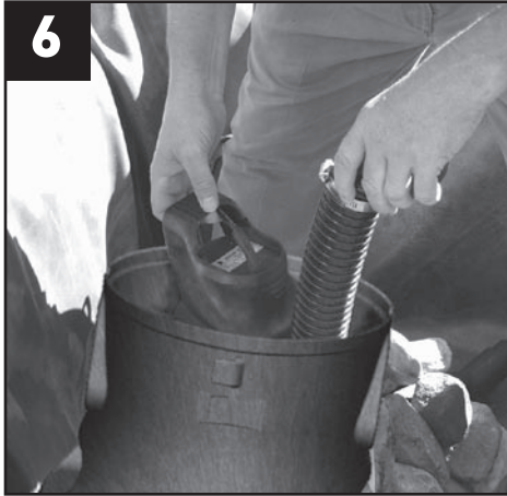
Lower pump into Waterfall Well.
