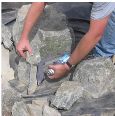
Use expanding foam to fill in voids between rocks.
