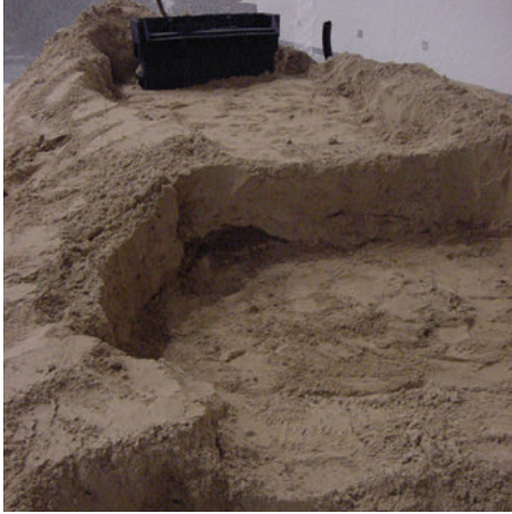
Sculpt dirt in stream area before installing liner
