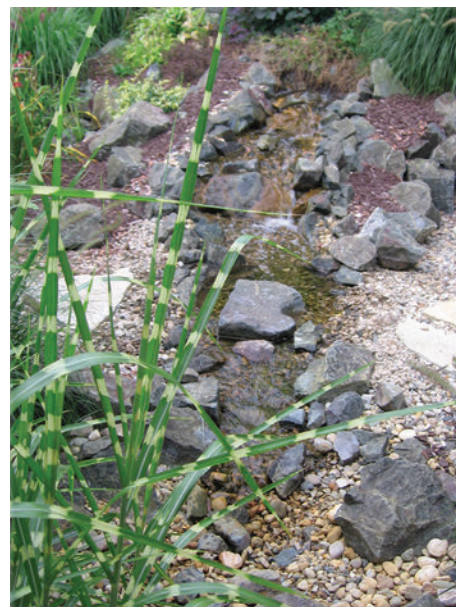
Once large rocks are placed and any foam work is done, sprinkle 1"-2" stone over stream rocks to fill in voids and cracks.
