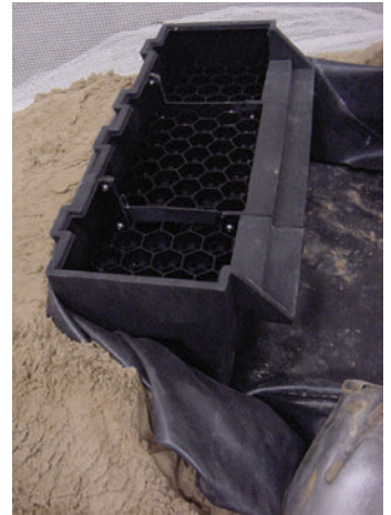
The liner goes under the spillway and wraps up the back and ends.
