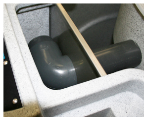
Figure 17.3 - By-pass in operation
