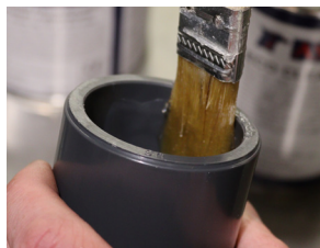
Apply glue to inside and...
