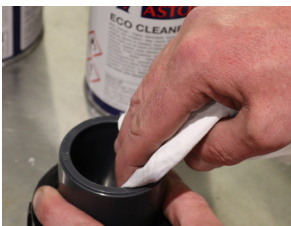
Clean pipe first
